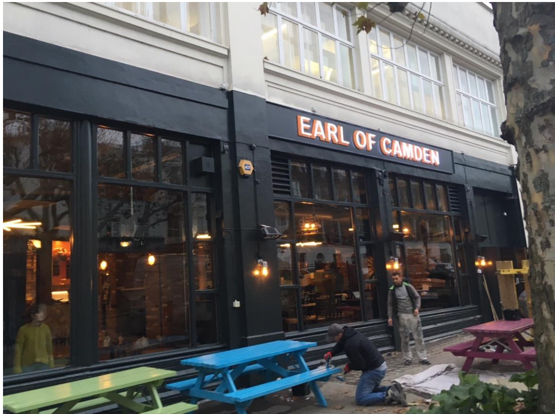
1. Albert Street Elevation showing signage and lighting
