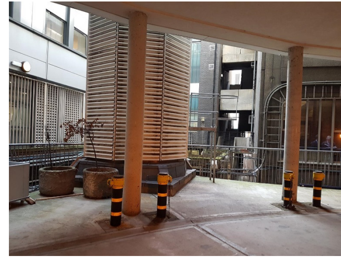
▲ photo F: existing plant tower
