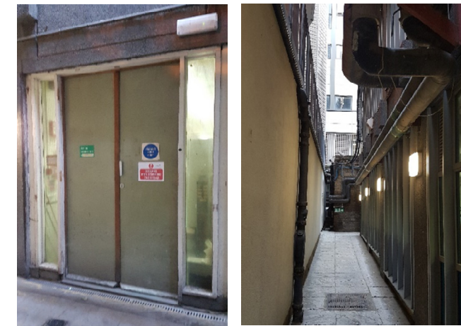
▲ photo K: existing doors
