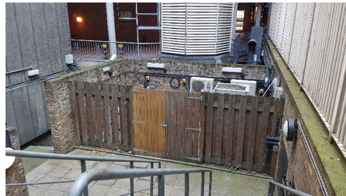
▲ photo B: existing rear plant compound
