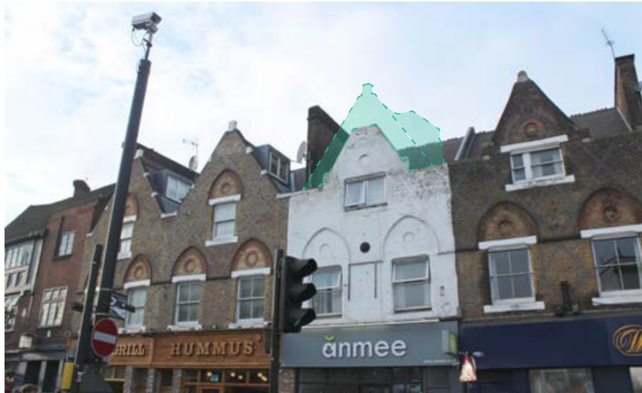
Existing view looking east along Camden Road
