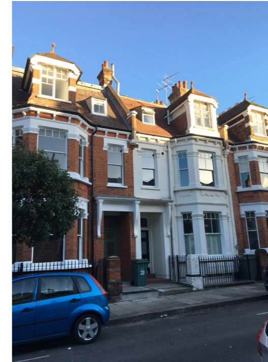
View of front of 18 Inglewood Road, existing front roof section to be preserved as existing
