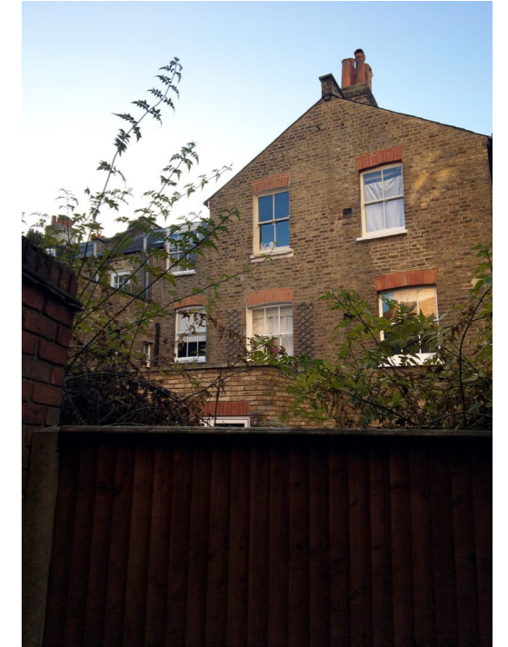
View of rear of 18 Inglewood Road. Access is not possible beyond this point.
