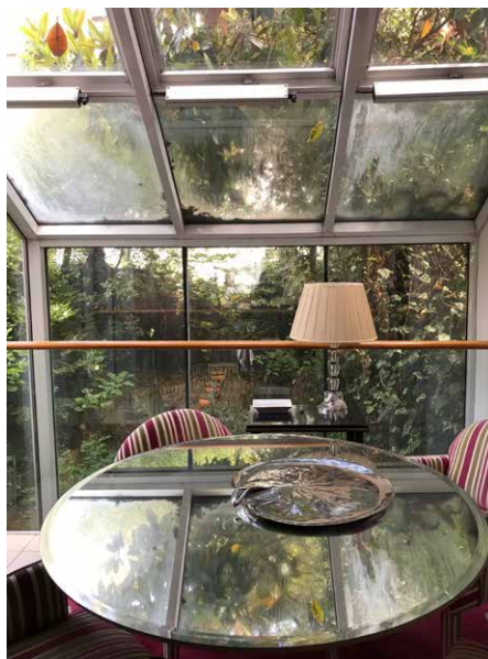
fig 12. Interior view of conservatory from ground floor - Note failing glazing and eaves position
