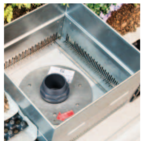
... depending on the type of retention spacer, the System Build-up “Stormwater Management Roof” retains a minimum of 80 l/m on the roof.
