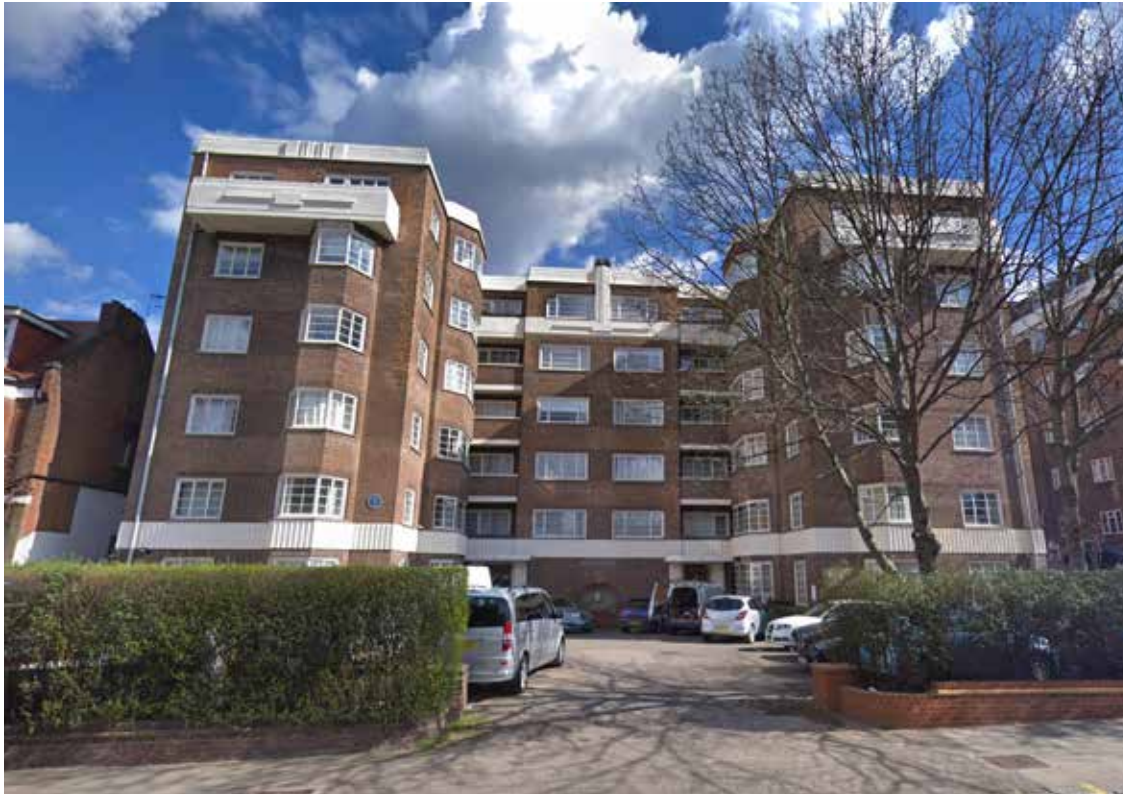
fig 3.11 Kendal Court on Shoot-up Hill showing central vehicle and pedestrian entry into site
