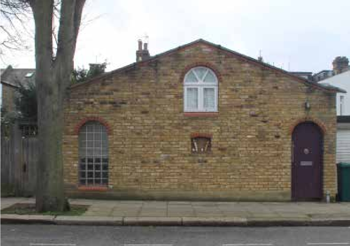
fig 2.5 The only residential (assumed) structure opposite the appeal site.
