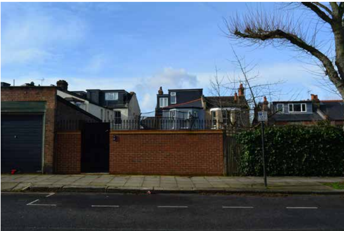
fig 1.4 View of rear accesses/garage opposite the reservoir site on Gondar Gardens
