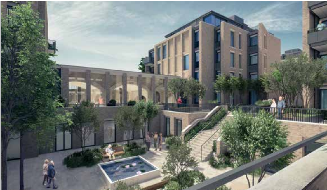
fig 3.18 View into street and lower courtyard, across to retained reservoir arches within restaurant
