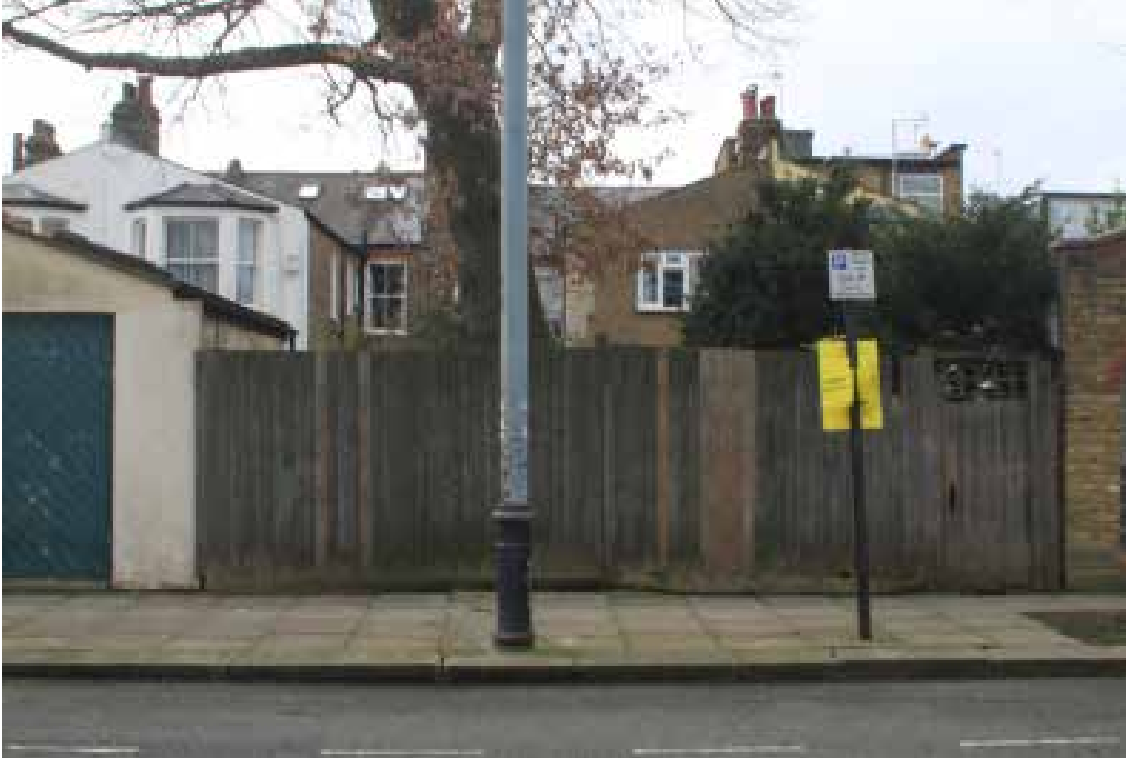
fig 2.7 Rear view of houses fronting Sarre Rd. This view is from Gondar Gardens showing poor street edge plus garages and planting frustrating overlooking on to this street from Sarre Rd buildings.
