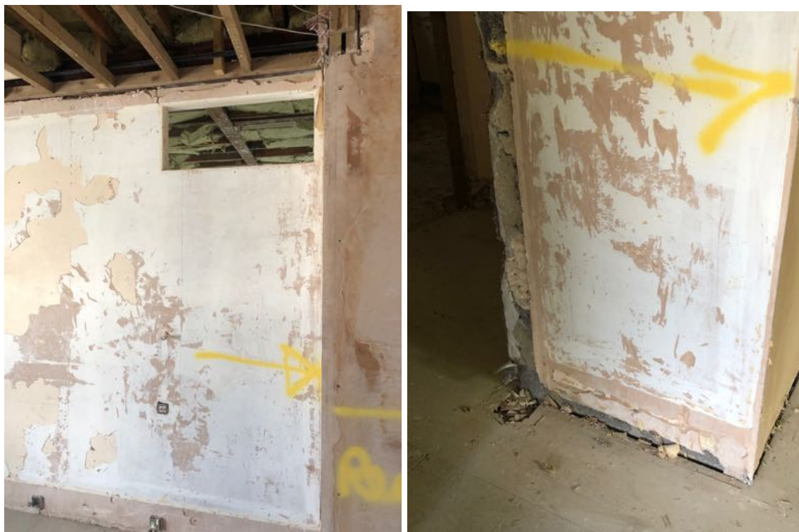
Figure 7 & 8: Modern breeze block and stud partition walls between the bedrooms
