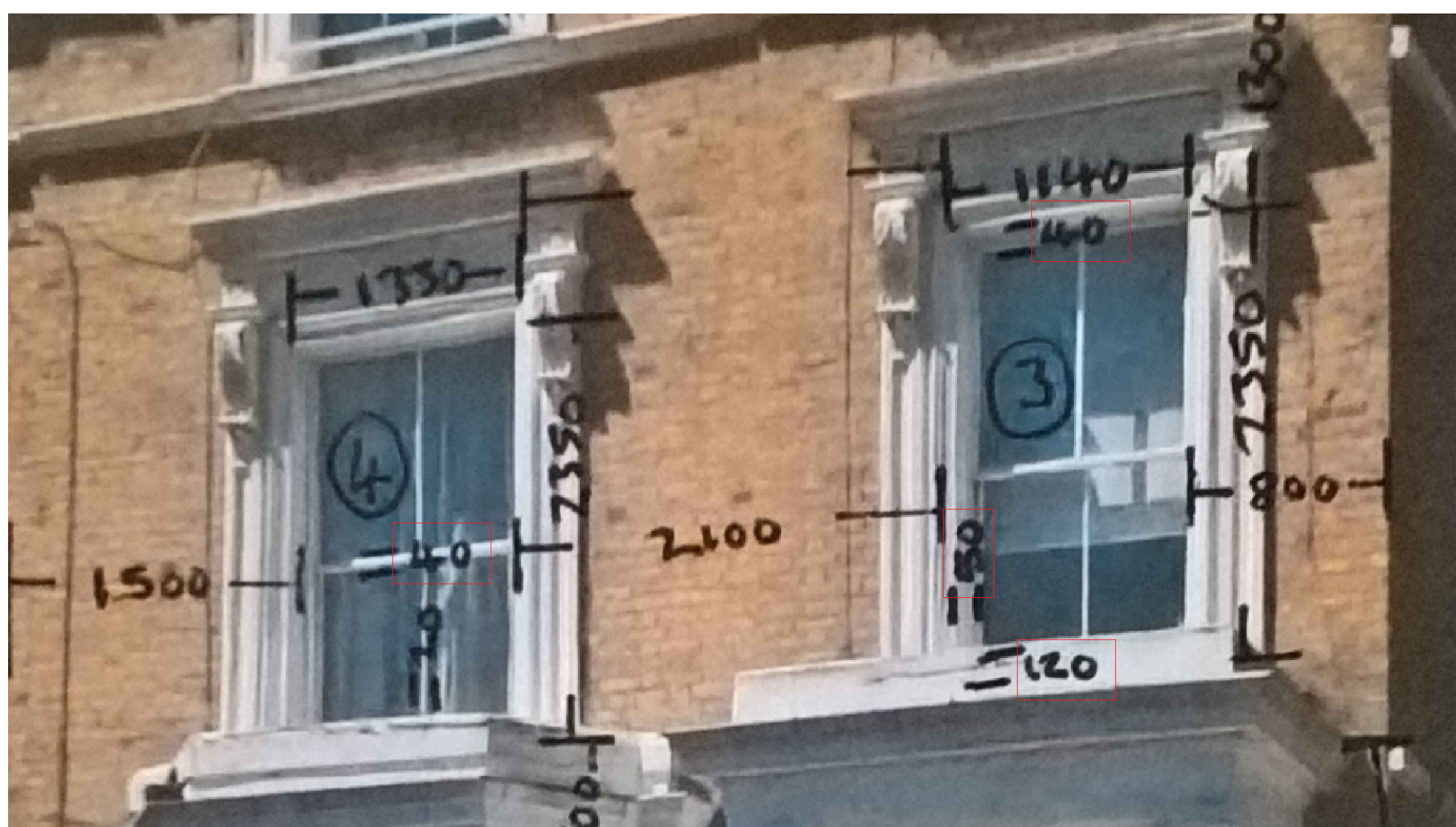
Image and measurements of the existing windows
