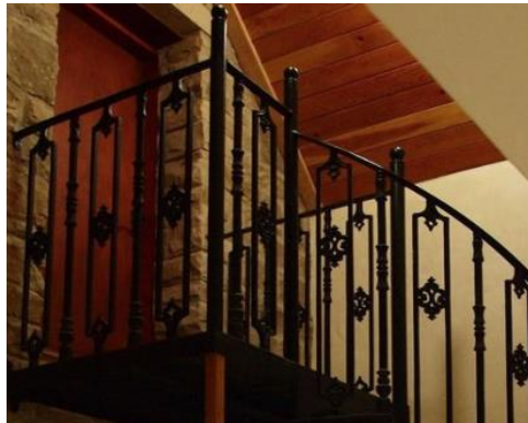
Traditional Victorian Railing
