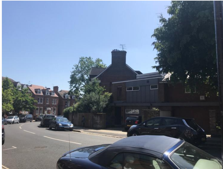
Fig 3 The application site looking east towards no.6 Hampstead Hill Gardens .
