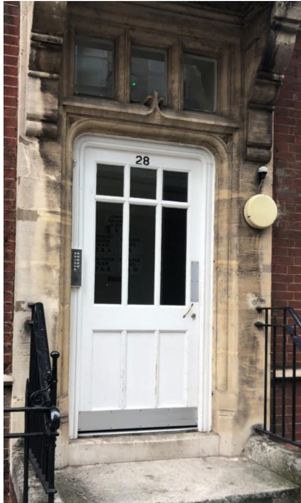
Photo of Front Door to 28 Longford Street
