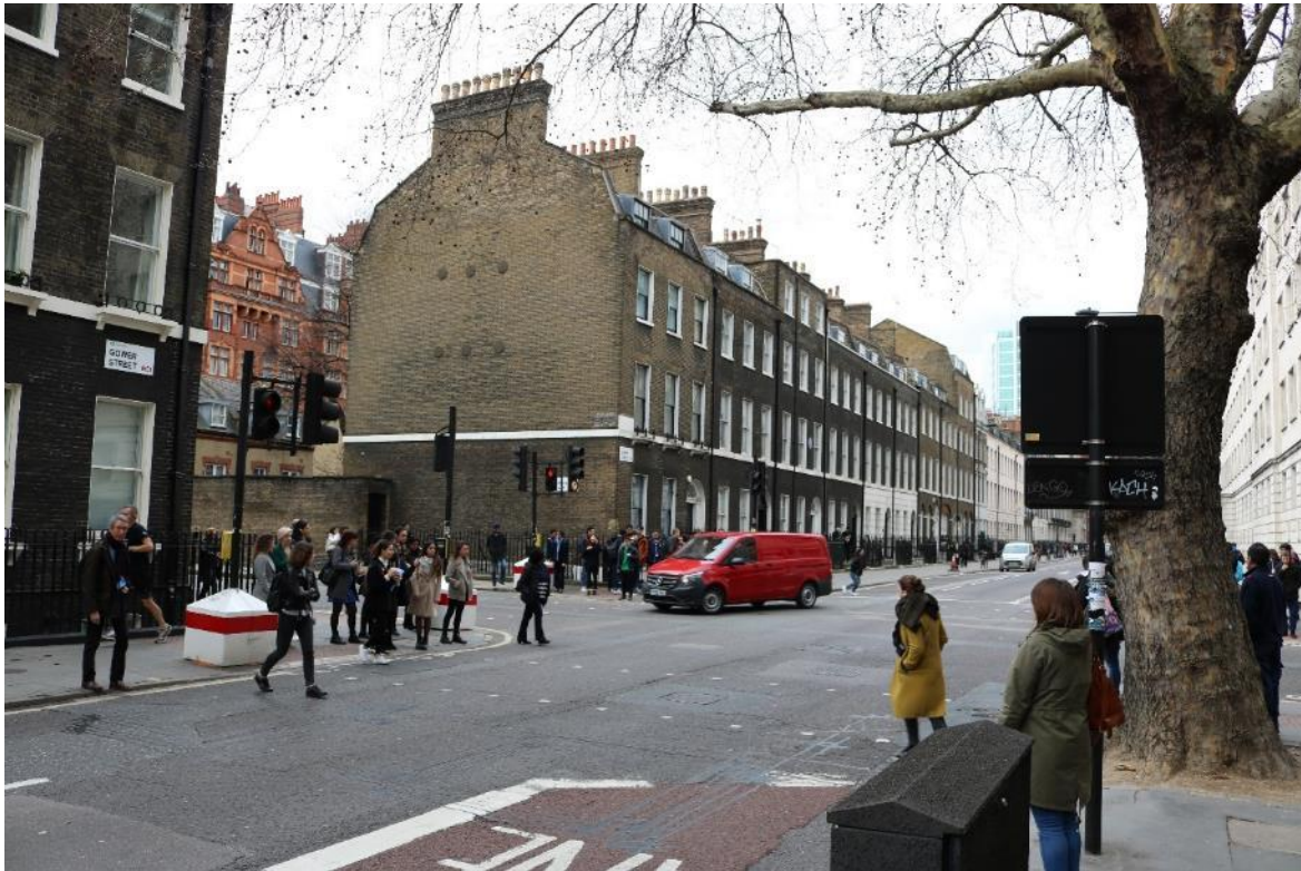
Image EDP 4: View of Number 87 from the south-east, showing the plain southern elevation and relationship with the rest of the terrace.
