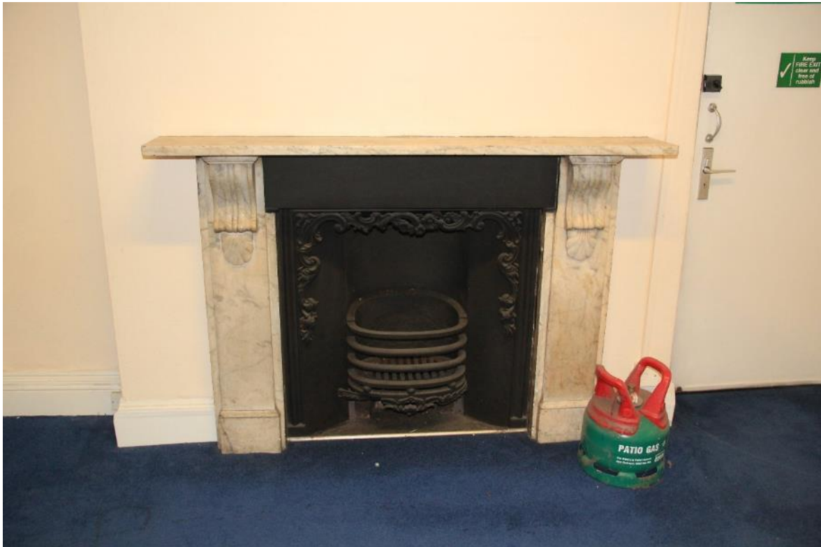
Image EDP 14: View of the fireplace in room G.2 looking south, showing its 19 th century style surround and grate. The door to the right leads to the later 19 th century porch add-on to create a second street level entrance.
