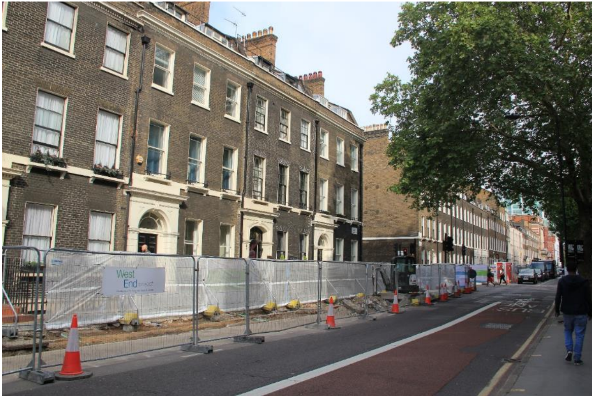
Image EDP 43: View of the terraces to the south of 87 Gower Street, looking north west with Number 87 appearing by the traffic lights. These townhouses are slightly more elaborate than 87 Gower Street, although they clearly demonstrate a unity of scale and character.
