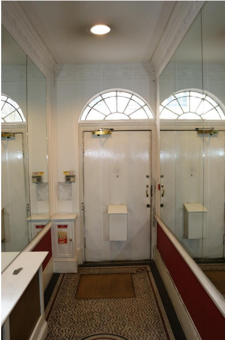
Image EDP 8: View of the entrance lobby G.1 looking east towards the entrance door. Note the decorative cornice and mosaic floor.
