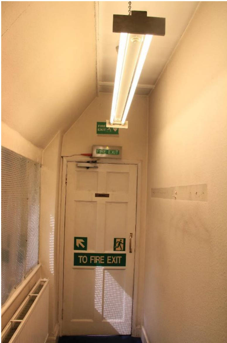
Image EDP 15: View of the corridor and modern partition in the rear extension looking west.
