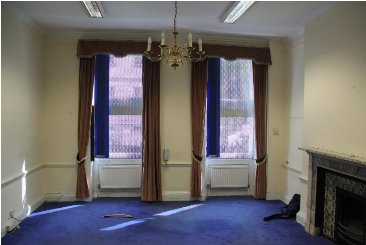
Image EDP 12: View towards the front (east) of room G.2 showing the window openings and fireplace to right.
