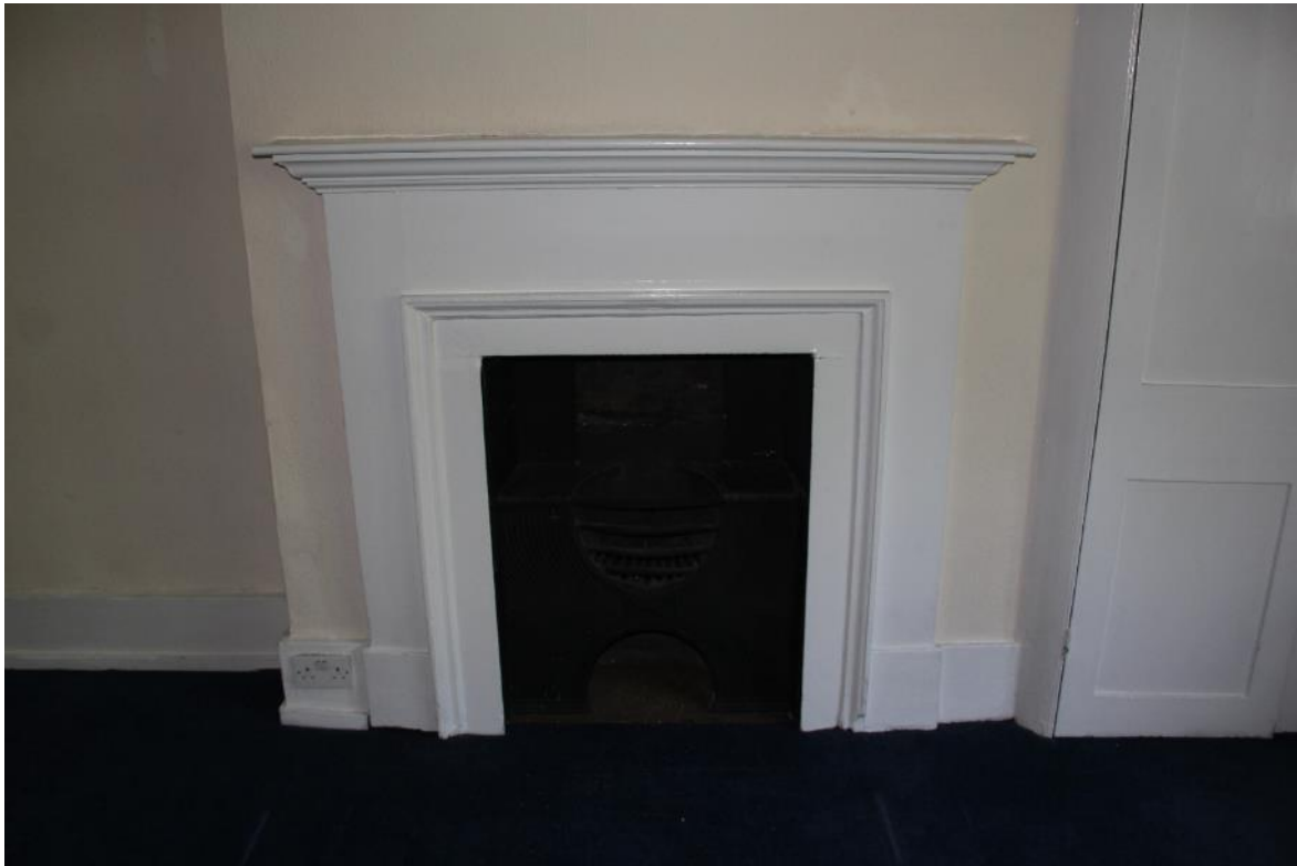
Image EDP 39: View of the late 18 th century style fireplace in Room 3.4.
