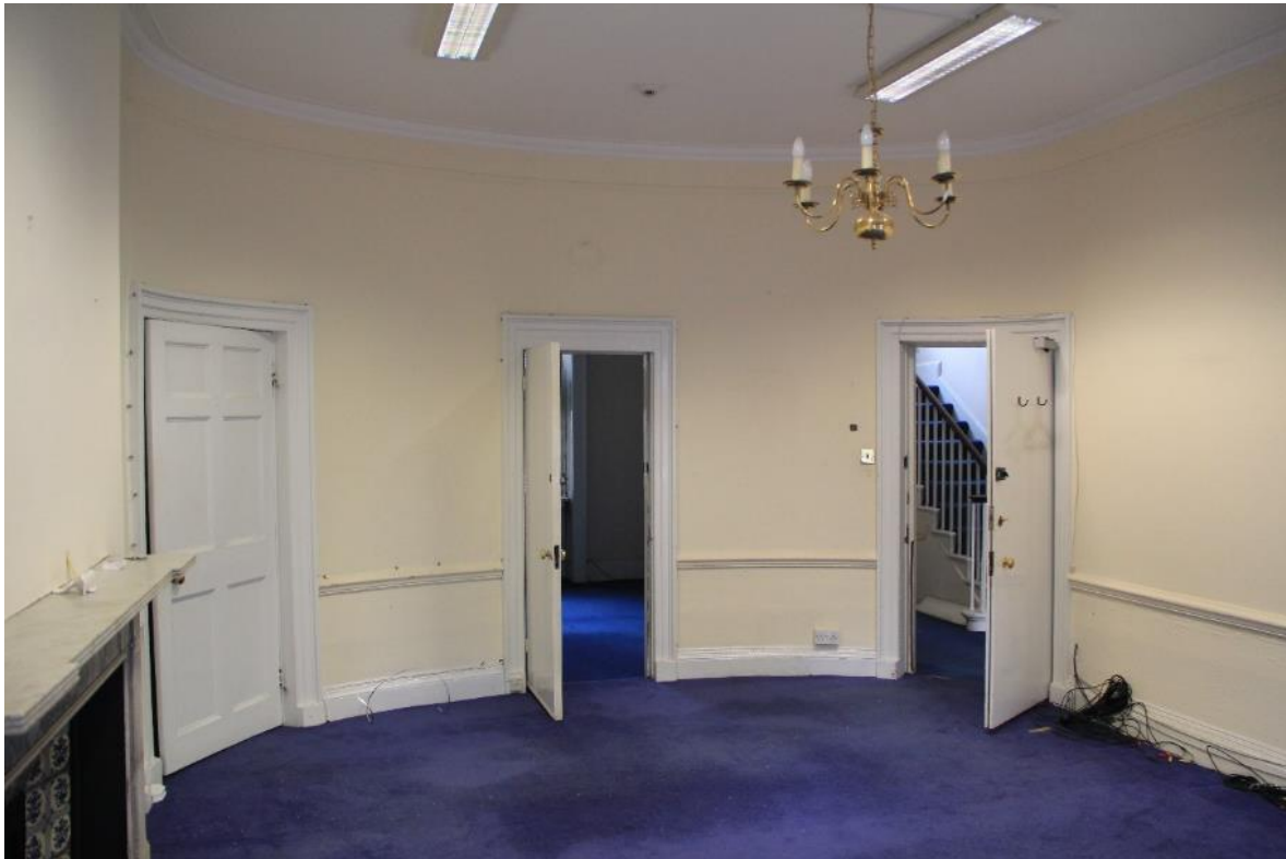
Image EDP 11: View towards the rear (western) wall of room G.2 looking west. Showing the characteristic curved wall at this end of the room. Note that the door architraves appear original, but the two main doors are modern; only the six-panelled door to the cupboard on the left is of original style.
