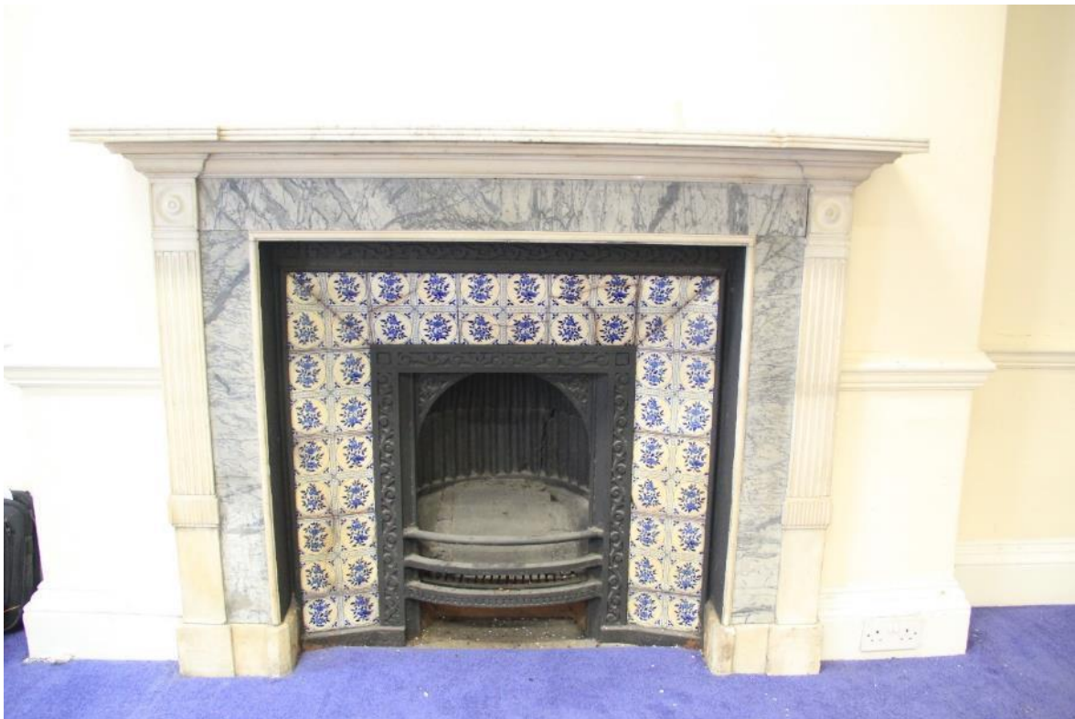
Image EDP 13: View of the fireplace in Room G2 looking south and illustrating the late 18 th century style surround and 19 th century tiling and grate.
