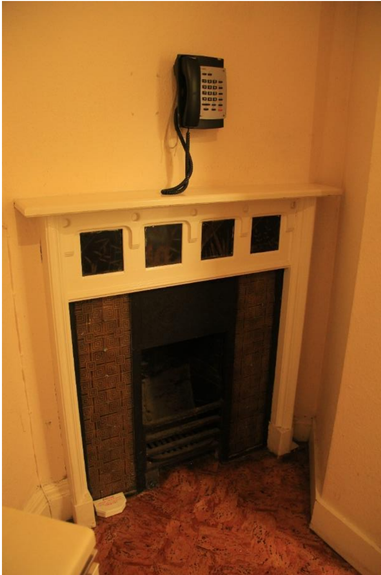
Image EDP 16: View looking east within the modern kitchen showing the inserted corner fireplace.
