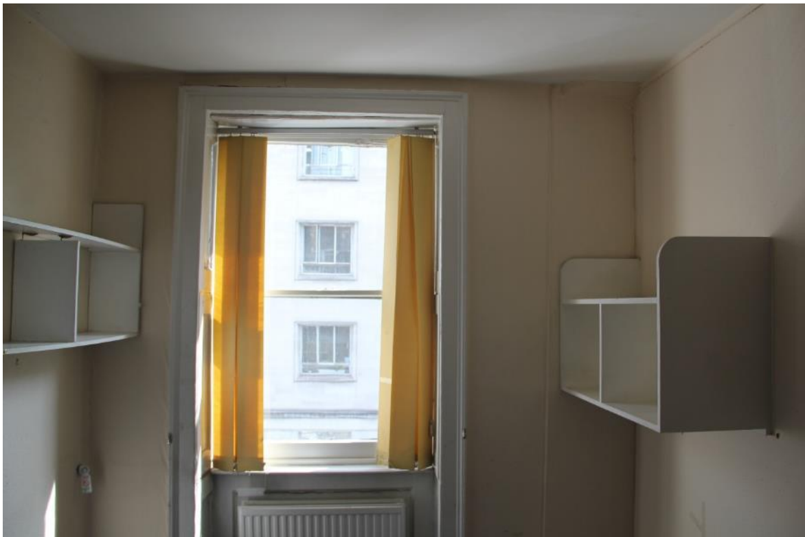
Image EDP 33: View looking east in Room 2.3 showing the cornicing to the top right continuing from Room 2.2. This demonstrates that the partition wall to right has been moved.
