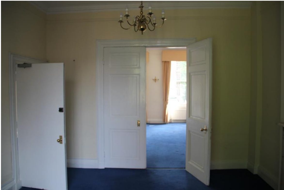
Image EDP 28: View looking east in Room 1.2 showing the 18 th /19 th century double doors and cornicing.
