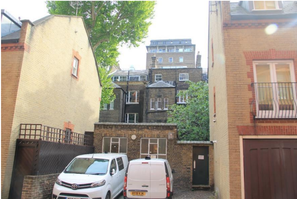
Image EDP 41: View of the rear of 91 Gower Street, looking east, showing the building occupying the rear space of this Grade II listed property that forms part of the same listing as Number 87. Also showing the full height closet extension not apparent on Number 87.
