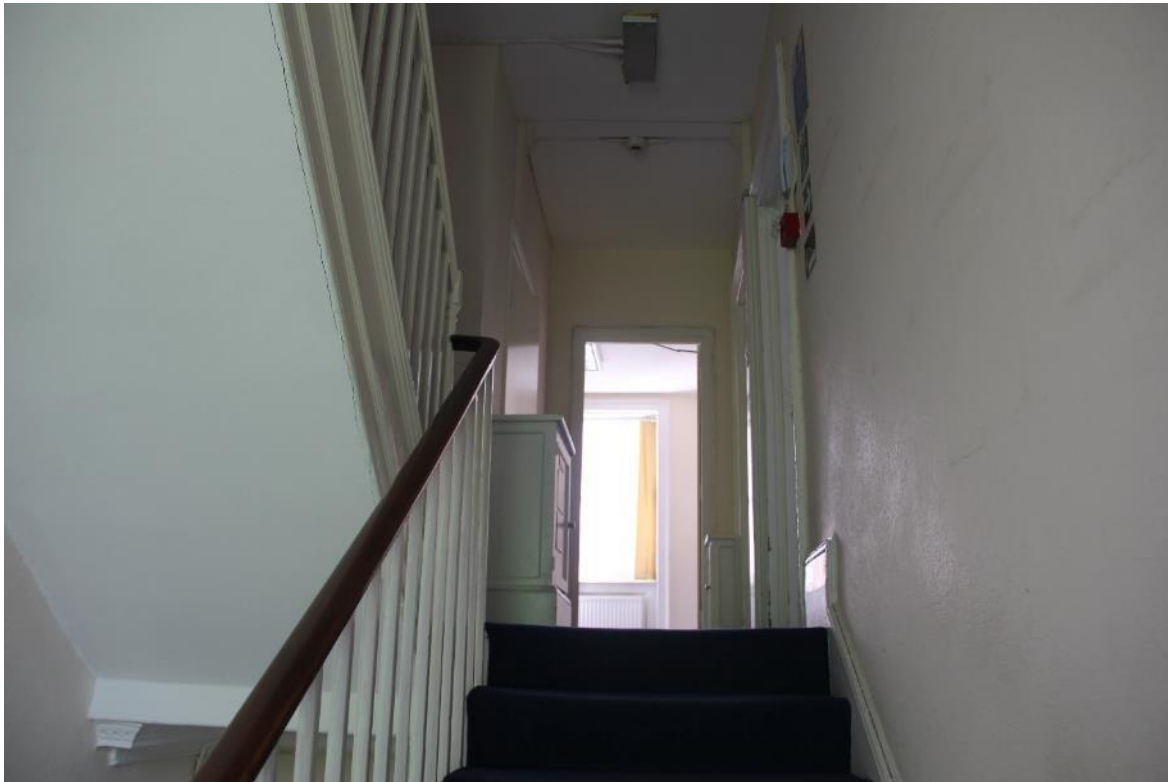
Image EDP 30: View east to the second floor landing. The ceiling has been dropped and the suggestion of springing points for a potential arch can just be made out. The inserted toilet can be seen to the left.
