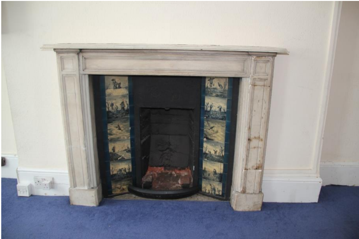
Image EDP 32: View of the fireplace in Room 2.2, with its Regency style surround and 19 th century inlay and grate.
