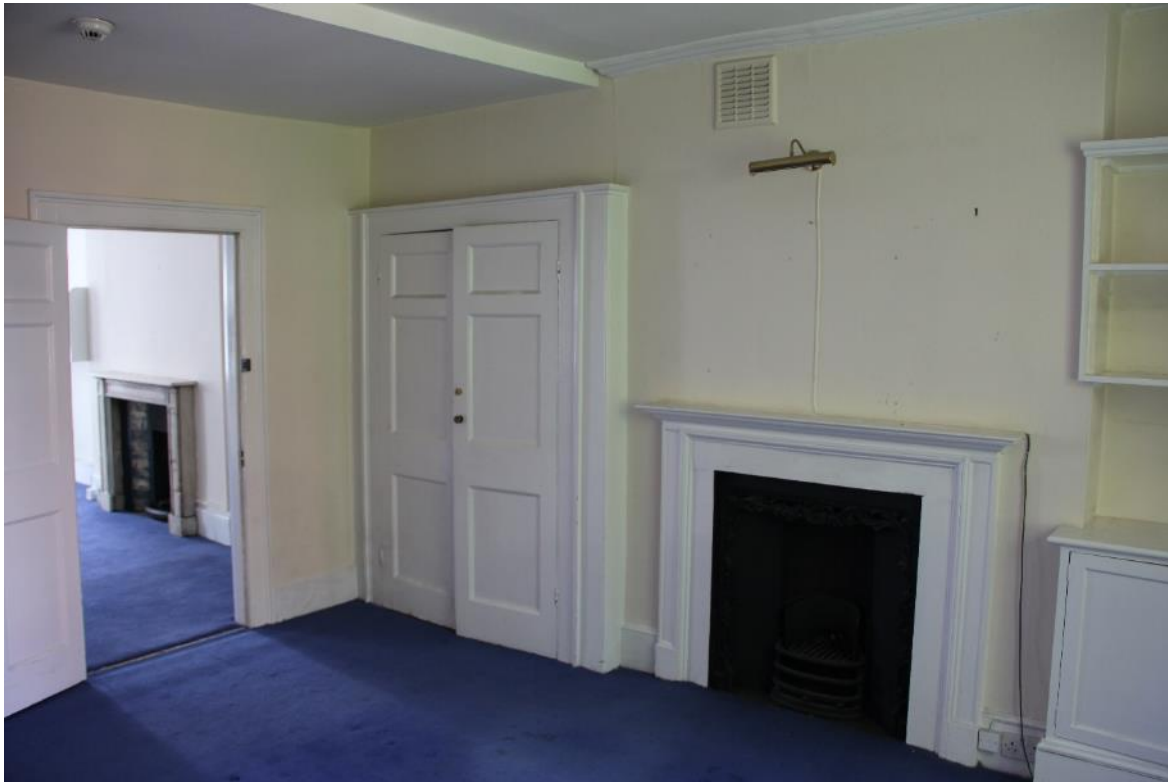
Image EDP 34: View looking south-east in Room 2.4, showing relatively plain timber fireplace surround and 19 th century grate. Also showing in-built cupboards to the left. Note the curtailing of the corning due to the dropped ceiling in the area, which also continues into Room 2.2 and the landing.
