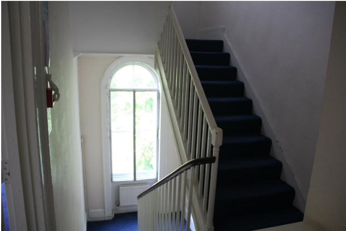
Image EDP 35: View west to the stairs leading up from the second floor landing to the third floor. Note the plainer style of handrail and balustrade, indicating that this leads to the servant's quarters at the top of the building.
