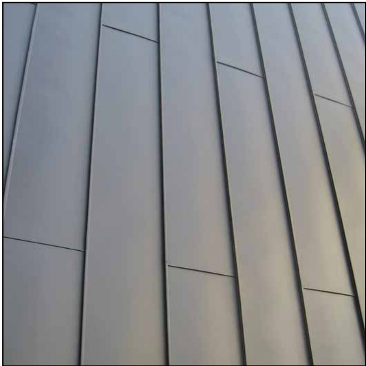
4 Zinc Roofing The mansard roof extension is will be zinc clad to integrate in the surrounding VM Zinc, Pigmento blue, Standing seam
