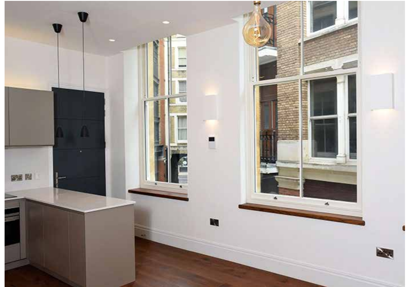
Example of a replaced Timber frame Sash Window
