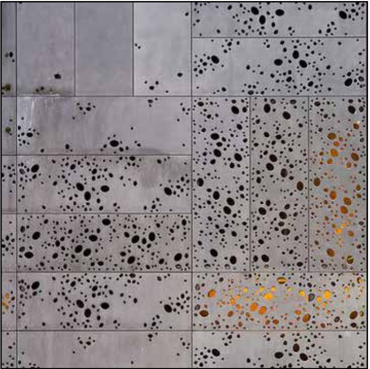
3 Decorative Metal Cladding Perforated metal cladding as transition from old to new brickwork Mapel Sunscreening Ltd, Aluminium Cladding, Powder Coating
