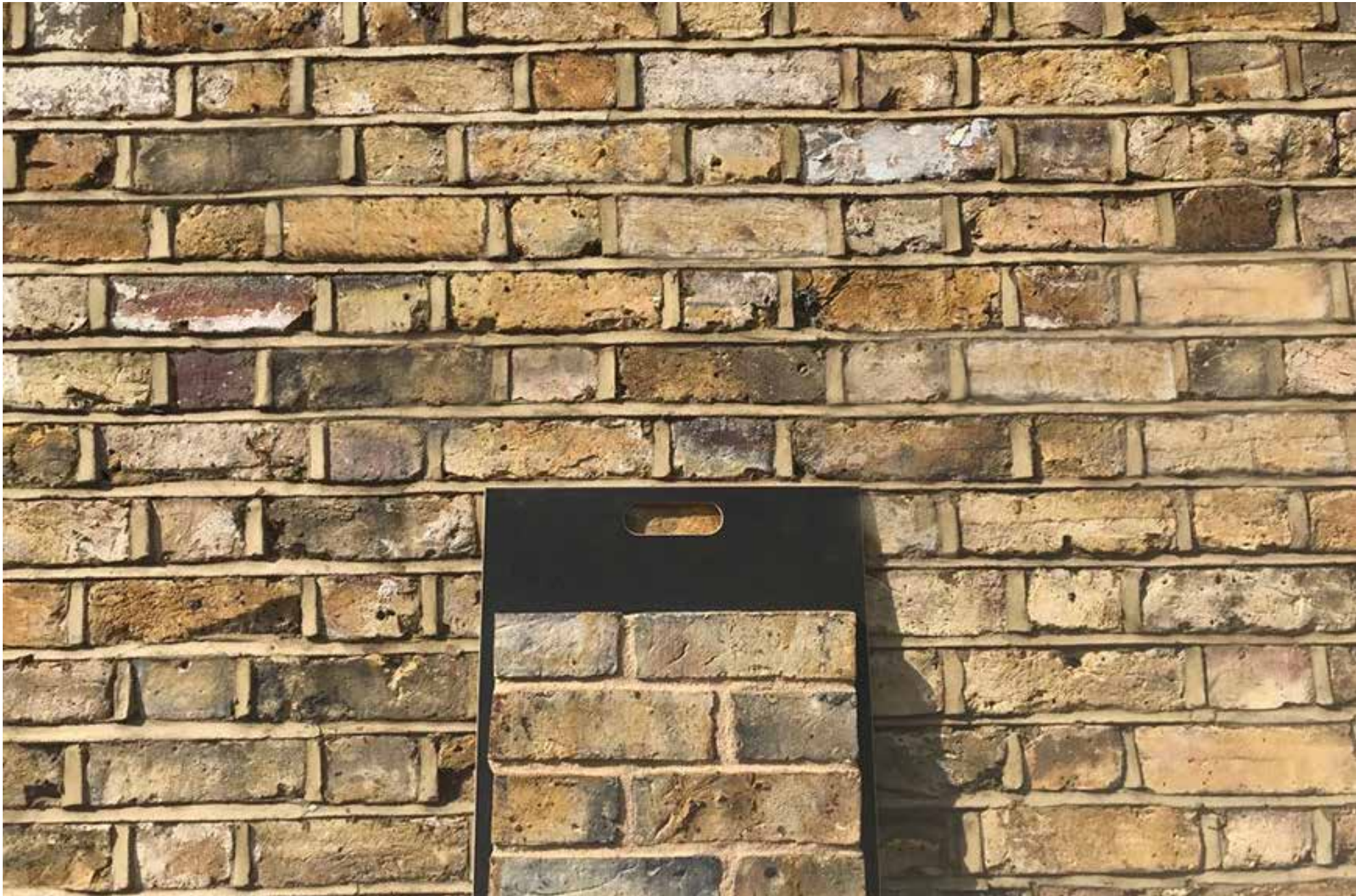
Example for matching London Stock Brick in front of existing Brick Wall
