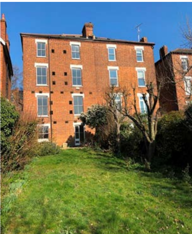
Rear elevation of No. 9 & No. 11 Nassington Road
