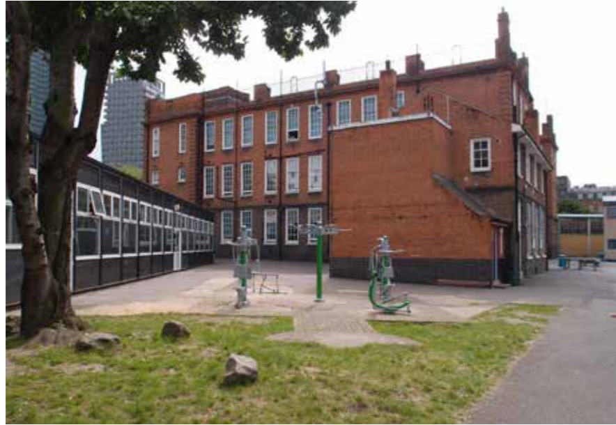
6 View of existing Maria Fidelis School and teaching portacabin from playground
