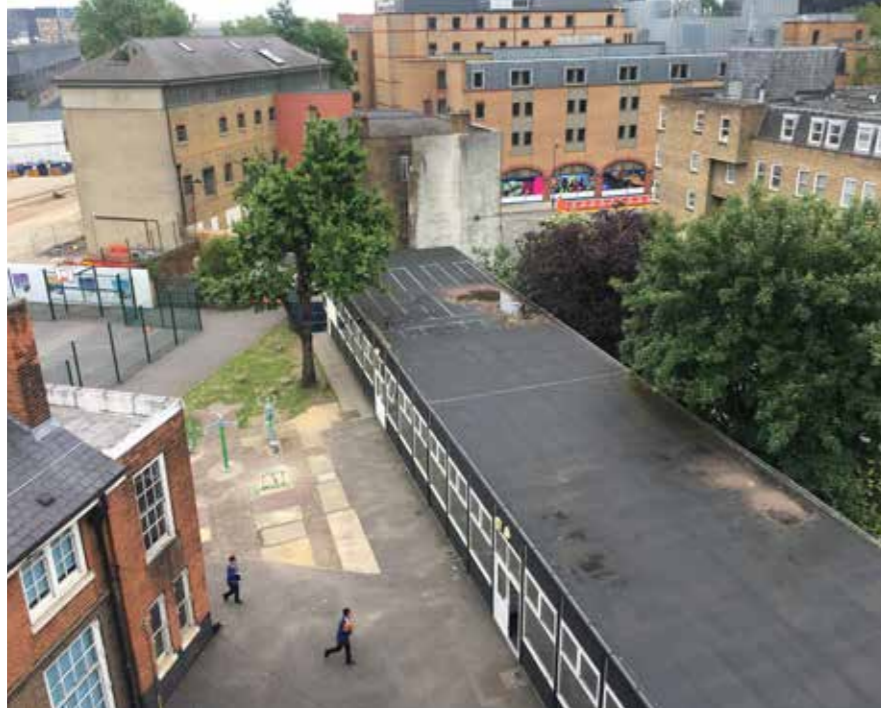
Cobourg Street buildings closed and soon to be demolished.
