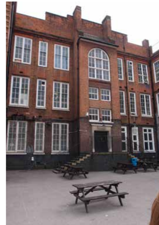
View of North Elevation
