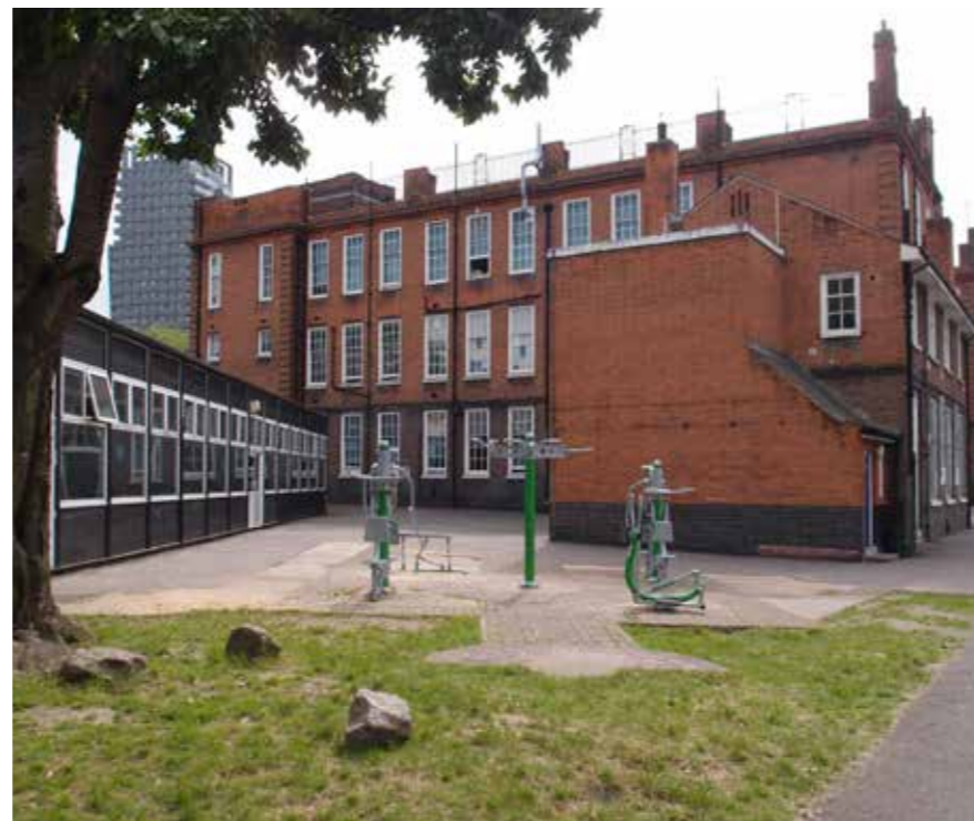
View of the 1950's extension and teaching portacabin
