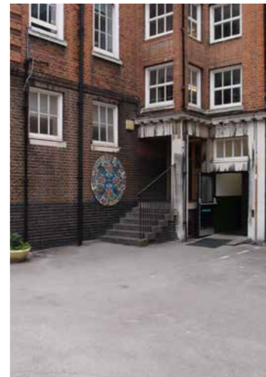
View of the current main entrance
