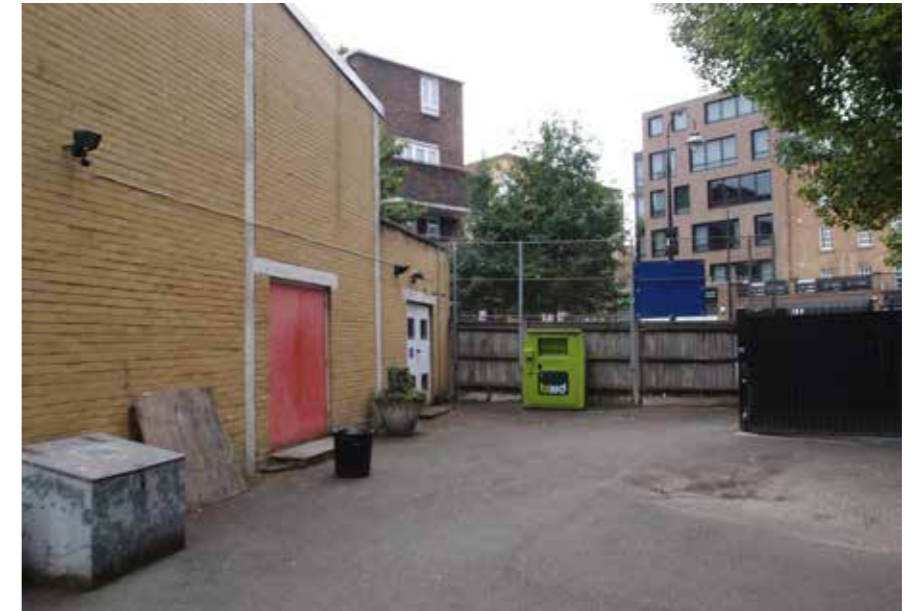
2 View of existing GYM
