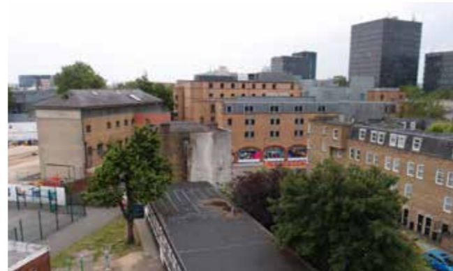
View towards Cobourg Street and Euston Station
