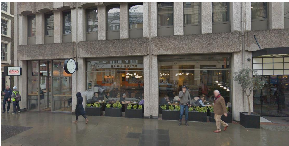
2. Coffeebar unit (now vacant), hotel lobby and entrance
