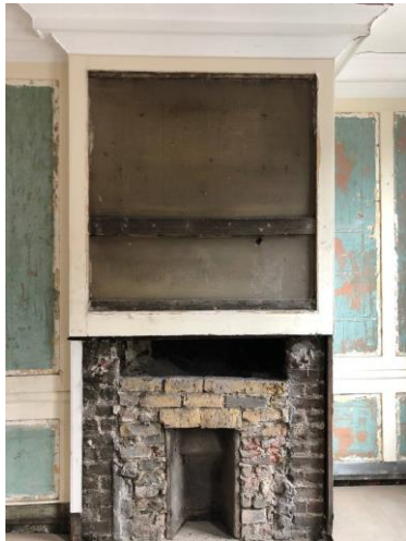
Figure 4. Second floor front room chimney breast.
