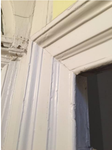
Figure 13 - image of original architrave from Great James Street
