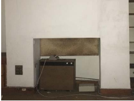
Figure 7 Existing lower ground floor front room chimneybreast
