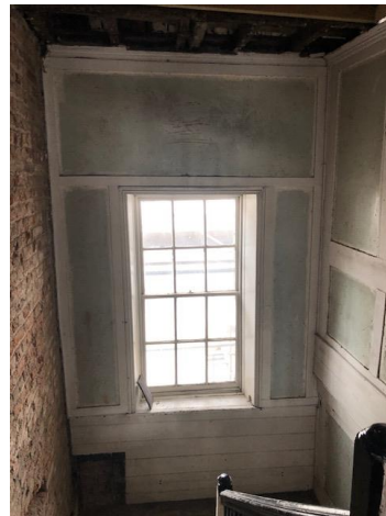
Figure 6. Third floor landing
