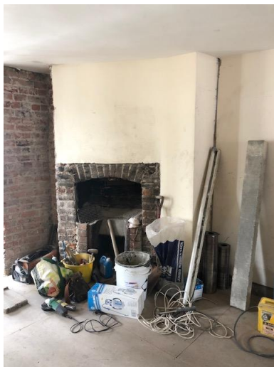
Figure 5. third floor rear room chimney breast
