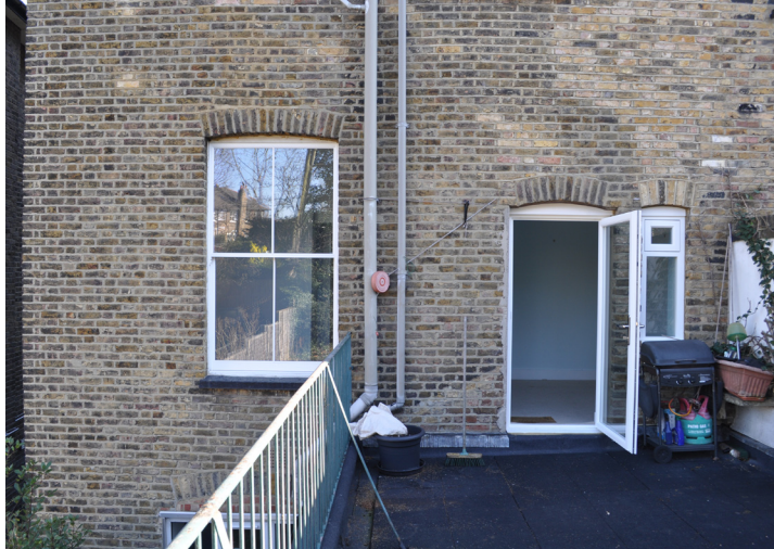
Right: Photograph of roof terrace area.
