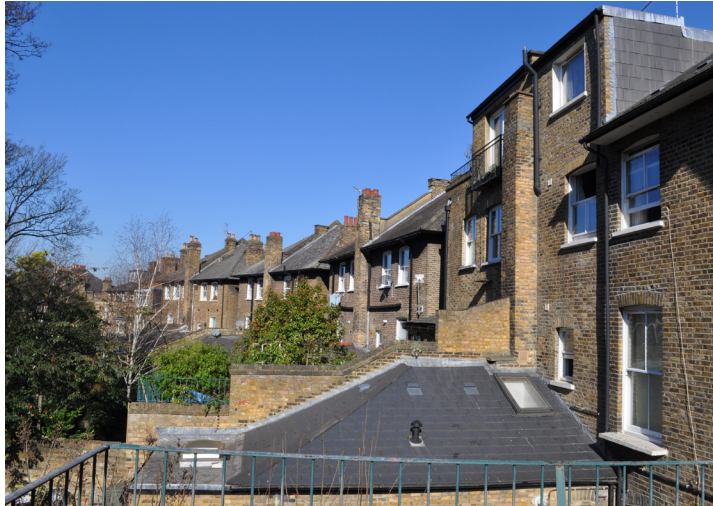
Right: Photograph looking north-west showing rear first floor extension at no. 149 Brecknock Road.
