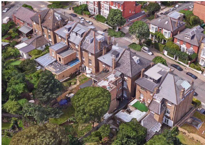
Right: Image from Google Maps showing various 1, 2 and 3-storey rear extensions on Lady Margaret Road.
