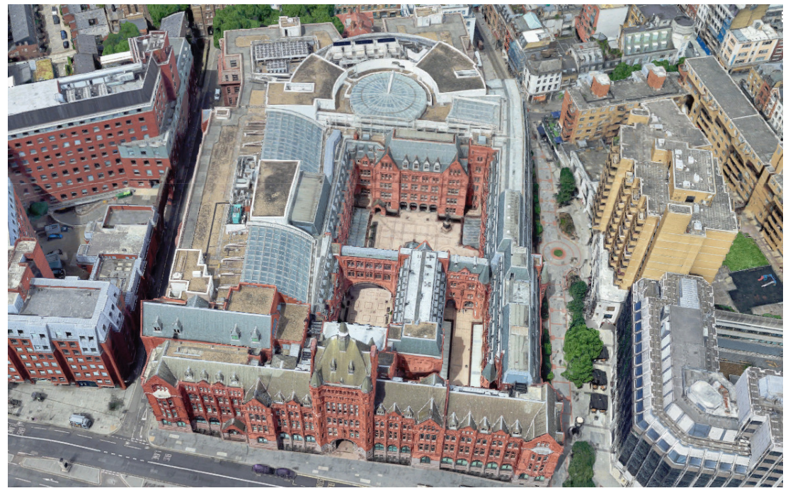
1 – view of building from South
