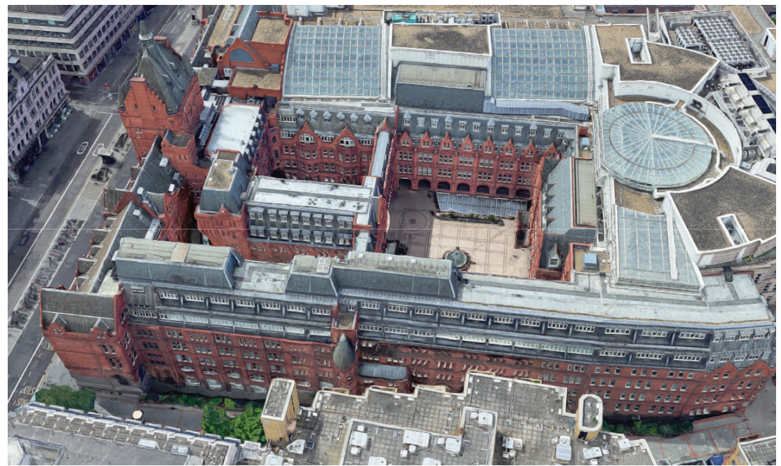
2 – view of building from East
