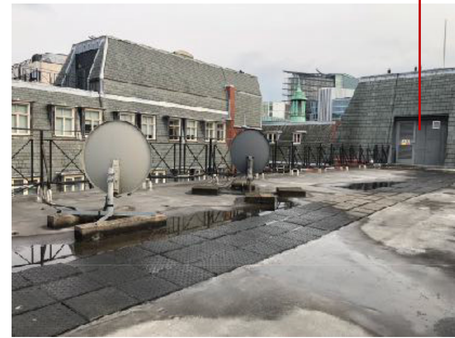
3 – roof showing existing satellites
