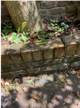
T2 physical damage to wall and pathway
