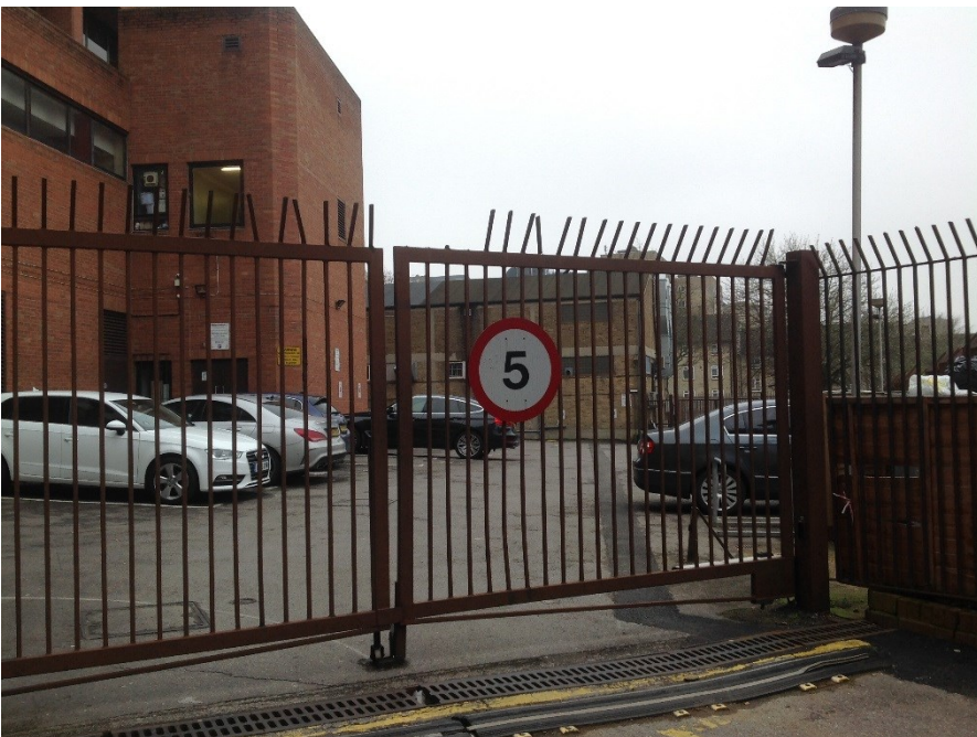
(3) Access into the car park to the rear parking area to 121 Finchley Road of locked with no access for delivery drivers
