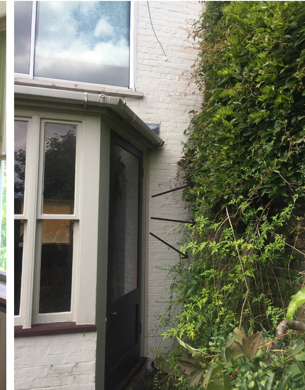
02. external view of rear access facing brick wall
