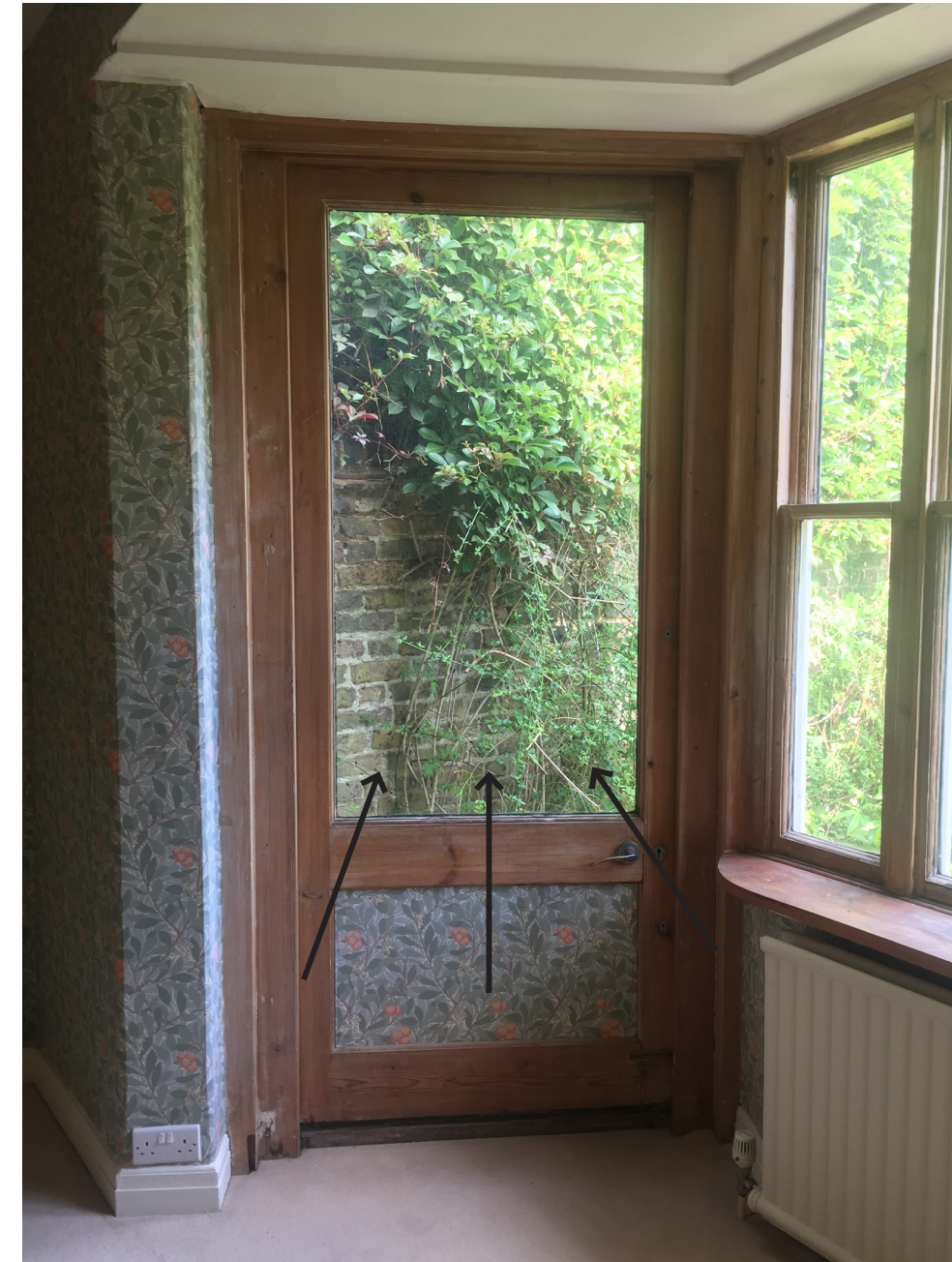
01. existing view towards brick wall
