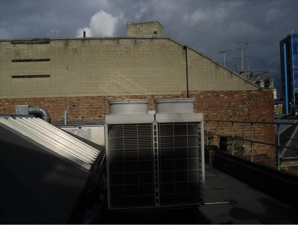
Flank wall of nos. 20 & 22 Stuckeley St./ Existing plant
