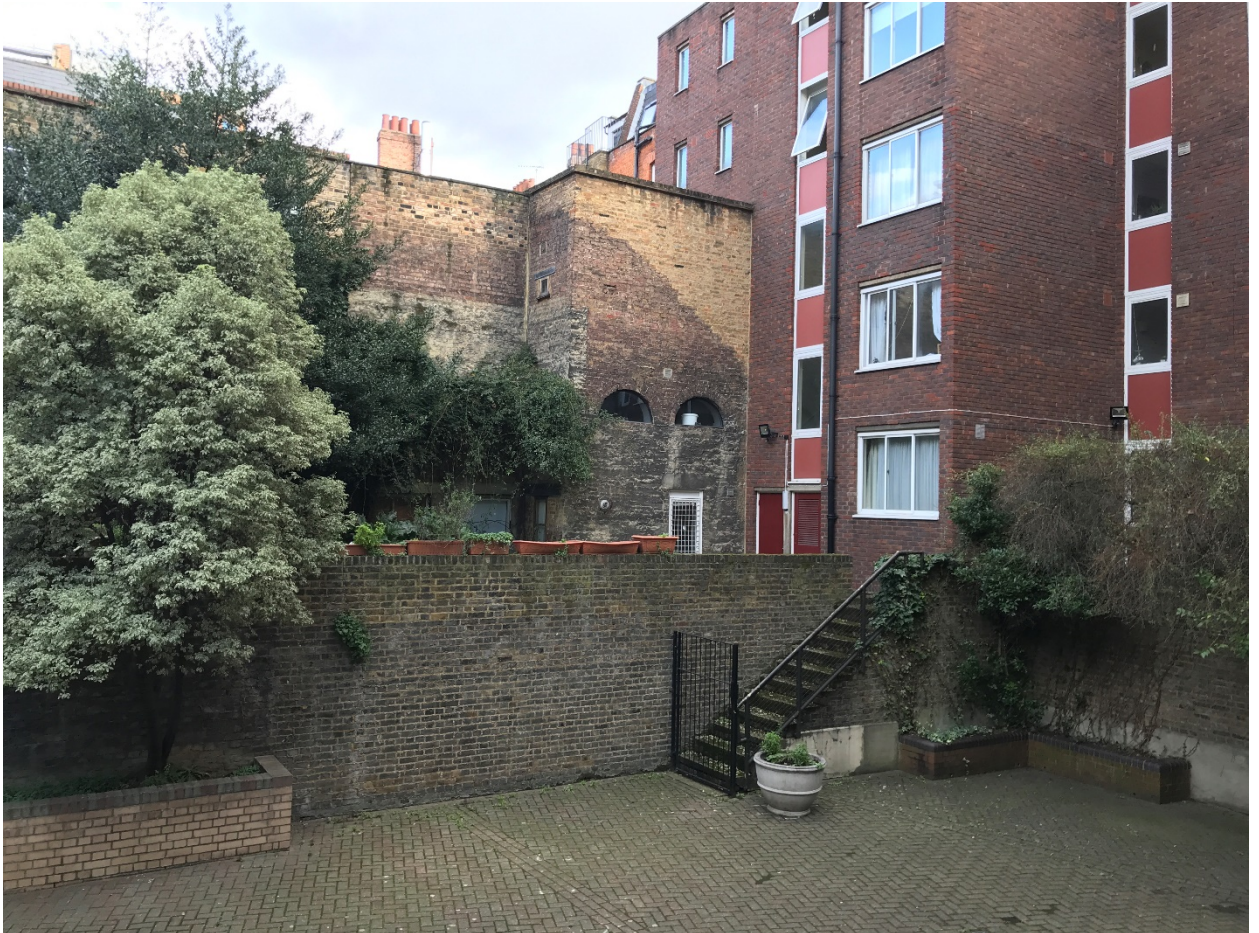
A2.4 Rear/West Elevation, showing crescent windows, built up wall and roof (lighter brick) above the 'absorbed' section of the former adjacent property.
