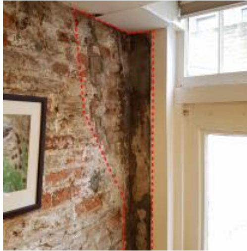
Figure 4a: Bed Joint – 7a Lambs Conduit
