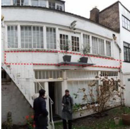
Figure 9: Spandrel Brick Panel
