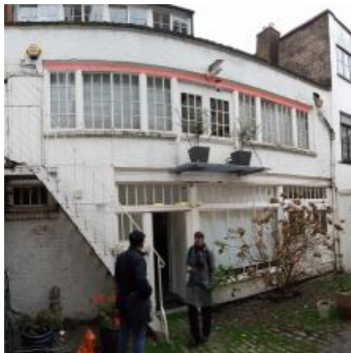
Figure 6: Second Floor Bressummer beam
