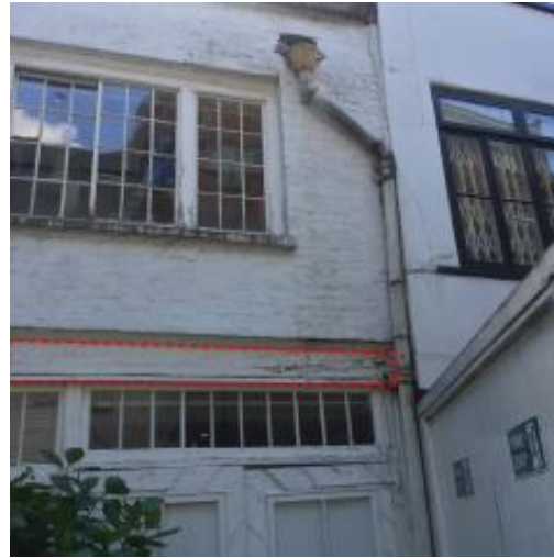
Figure 10: First Floor Lintel
