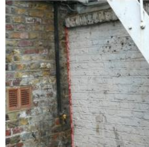
Figure 4b: Bed Joint – 18 Princeton Street side
