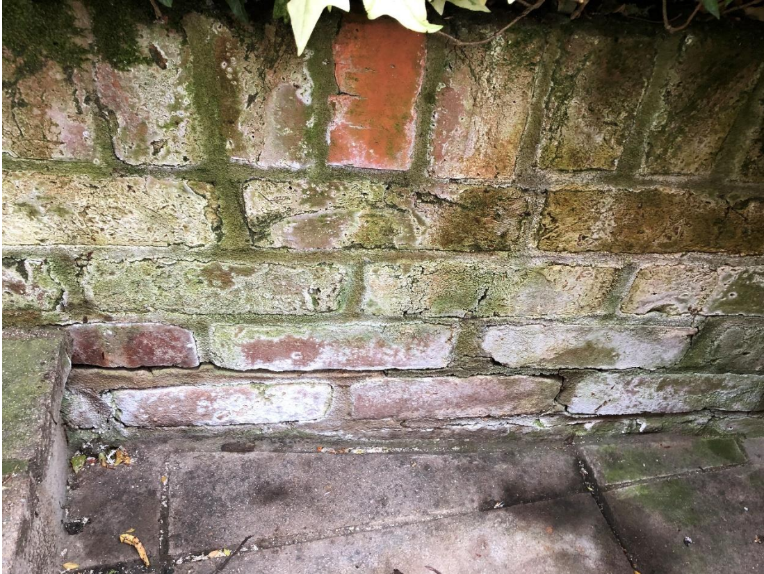
AEL-18129-PIC2 – Showing small crack in wall close to T.1
