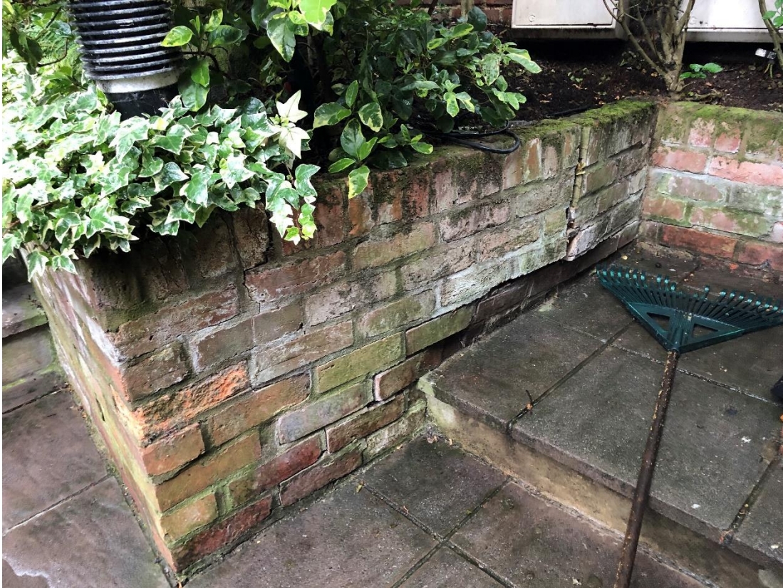
AEL-18129-PIC3 – Showing more significant crack in wall that will require repairing.
