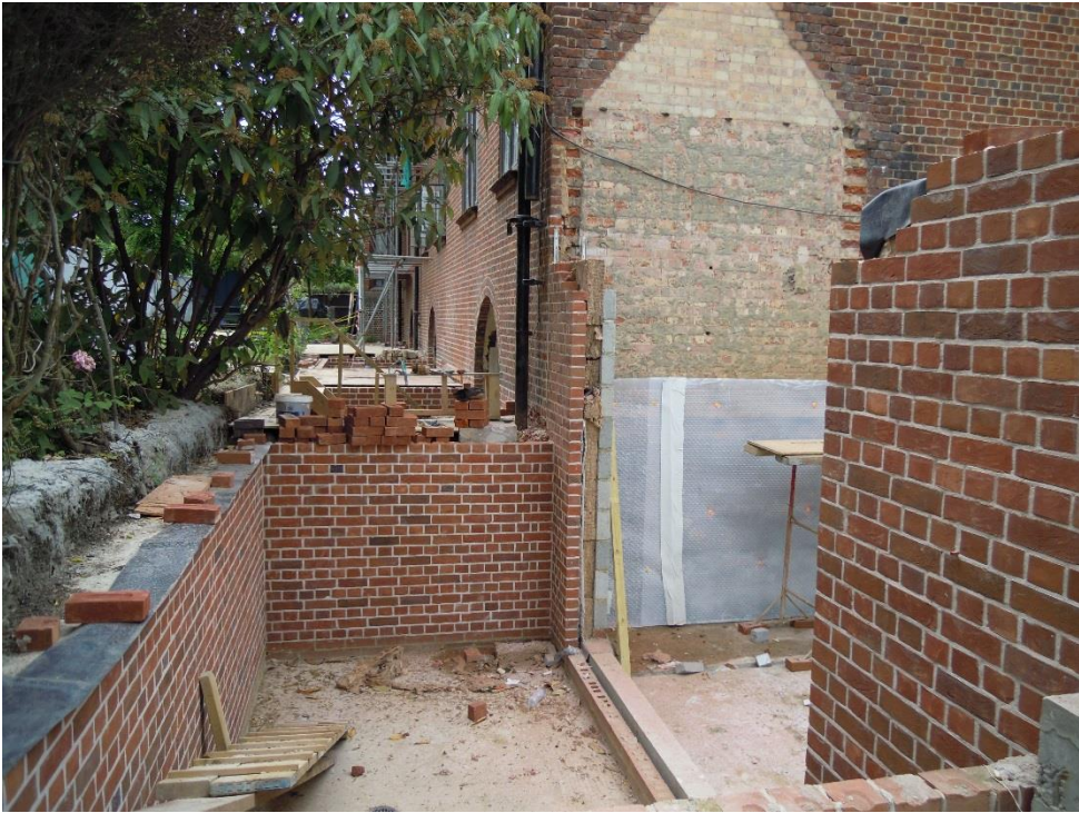
1. Rear elevation showing excavated lightwells
