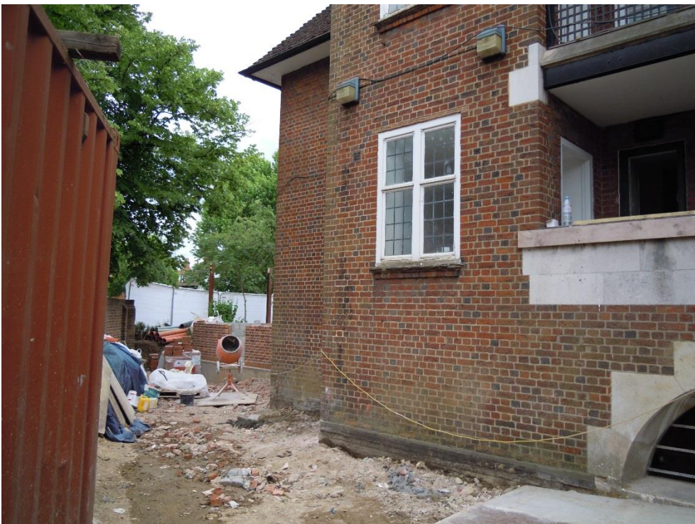
2. Front elevation showing side wing under construction
