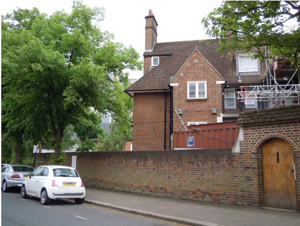
3. Front elevation from Lancaster Grove
