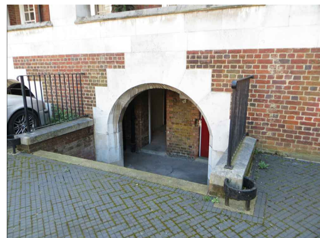
5 - EXISTING BASEMENT BALUSTRADE
