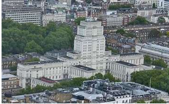
Figure 1: General view of the Senate House
