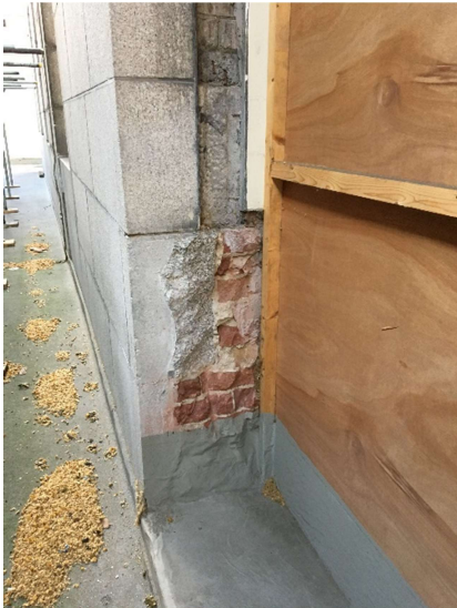
Figure 3: Current state of the openings
