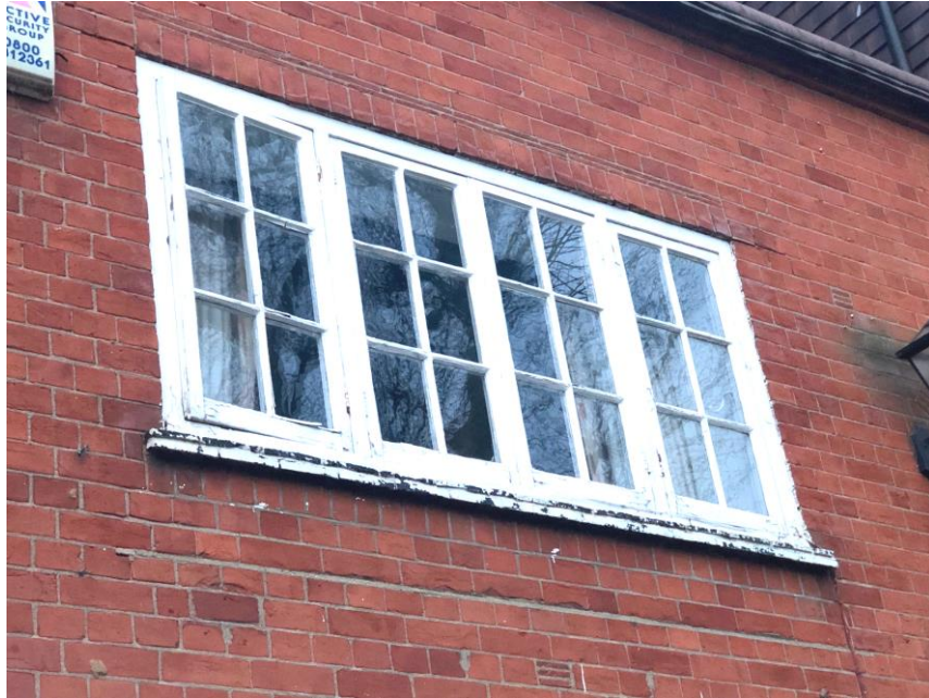
Figure 4. The close-up and wider elevation of the existing window at ground floor level on the front elevation with additional brick build up evident below the sill line.
