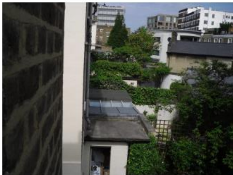
Single storey extensions at basement level
