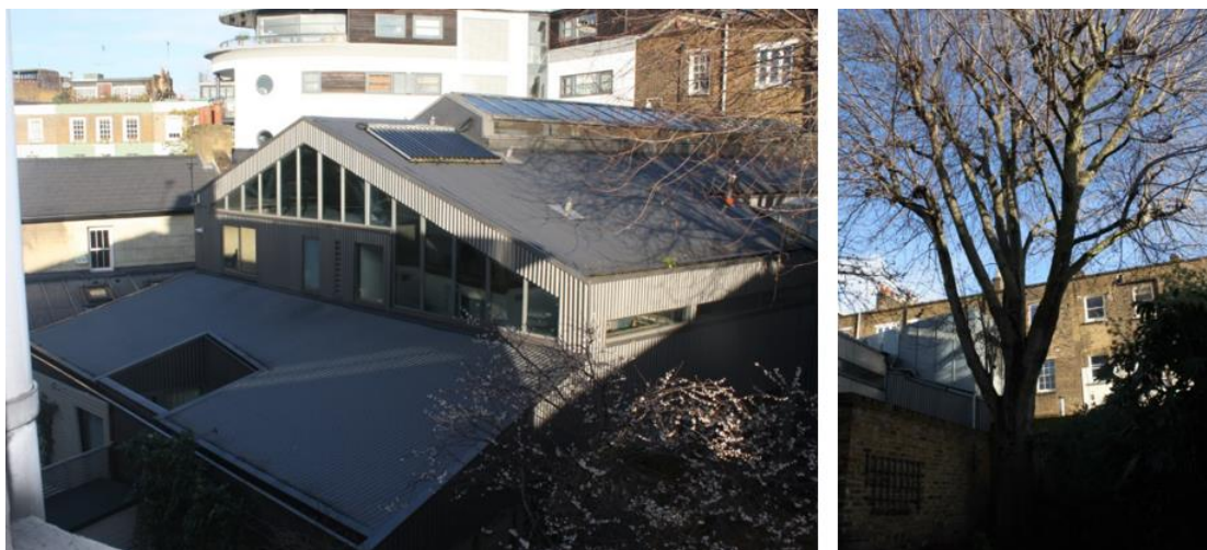
LIVE-WORK BUILDING (LEFT) AND SILVER MAPLE (RIGHT)
