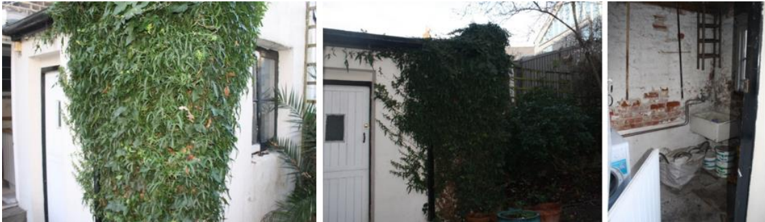
EXISTING REAR EXTENSION
