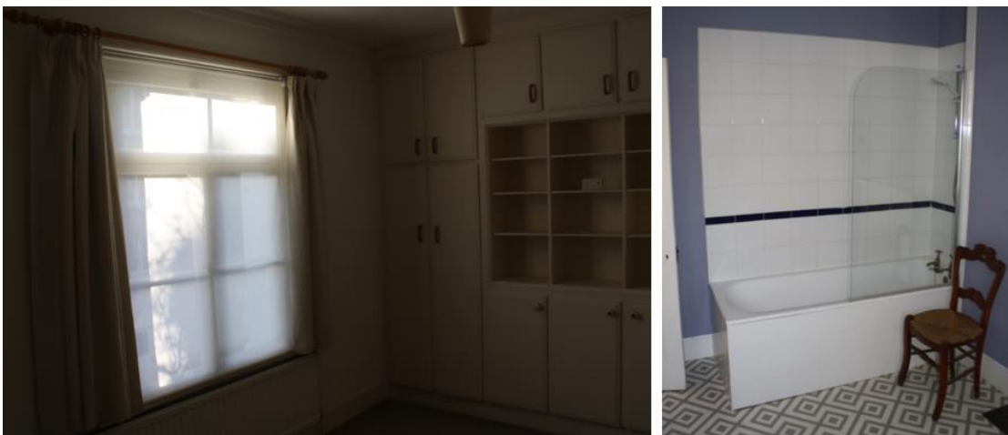
FIRST FLOOR BEDROOM AND BATHROOM
