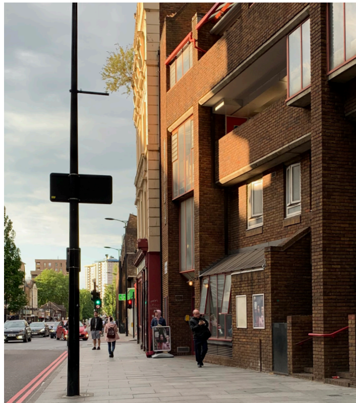
2 PHOTO OF EXISTING BUILDING
