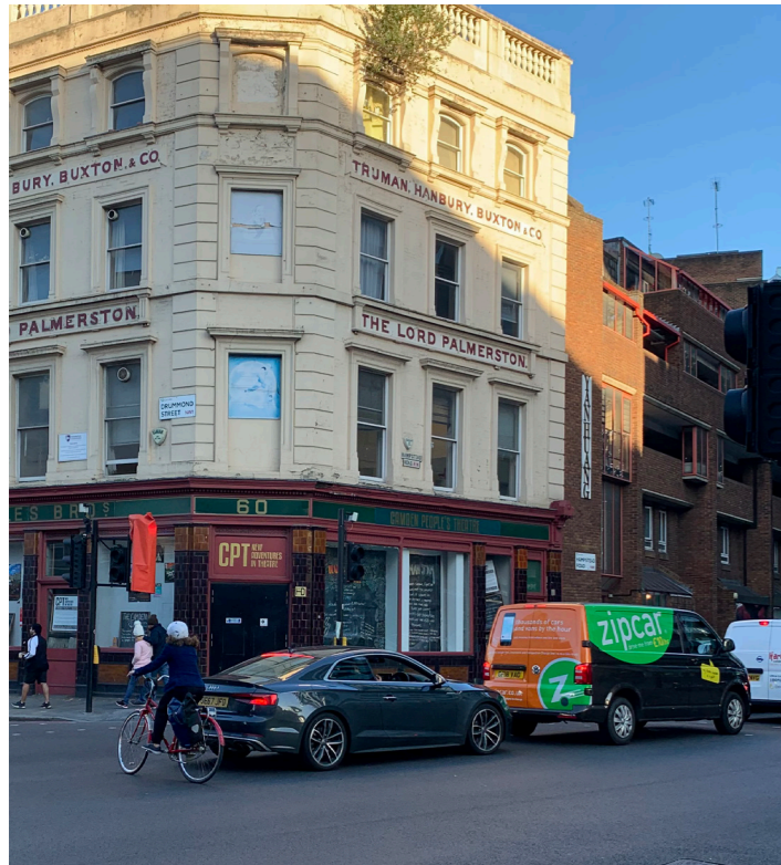
1 PHOTO OF EXISTING BUILDING
