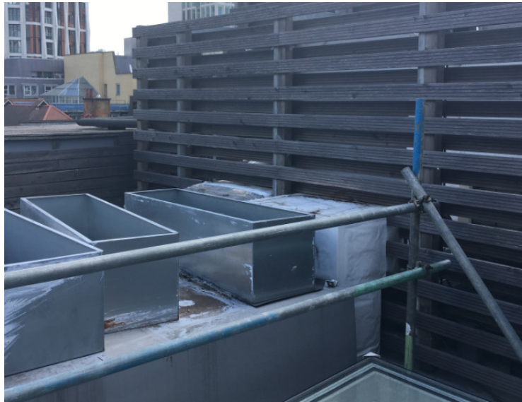
Figure 7: Existing plant compound screening (north-west elevation)
