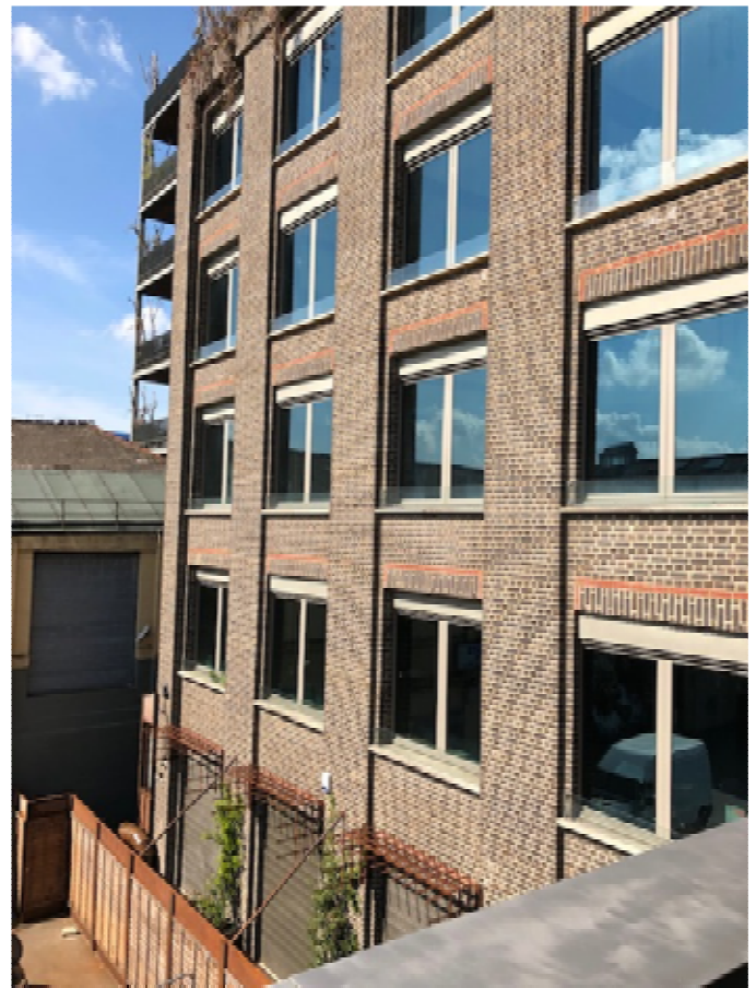
2) Rear elevation taken from terrace of no. 21 Ferdinand Street
