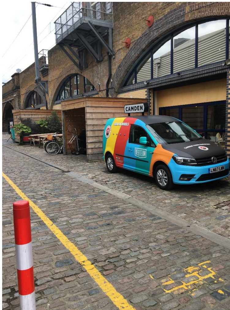
Image 8: View of tired storage sheds to be replaced with new
