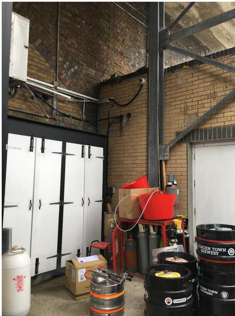
Image 4: View of storage yard to rear of Arch 55
