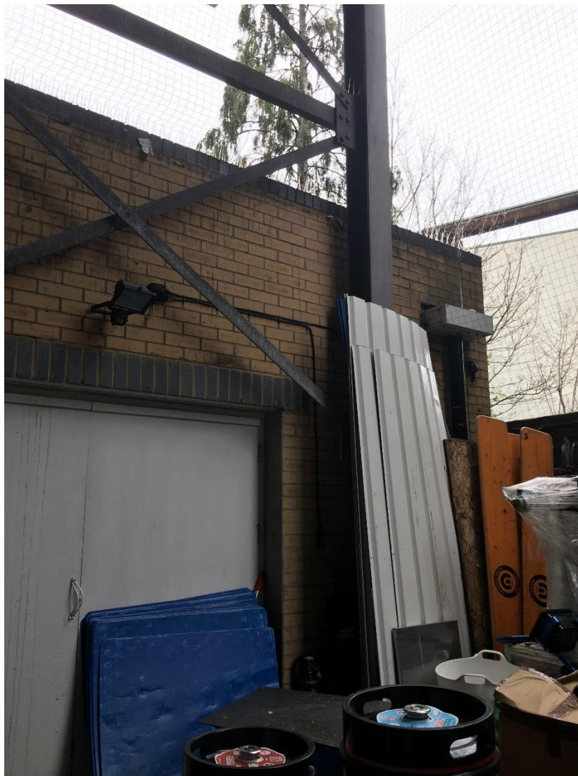
Image 5: View of storage yard to rear of Arch 55
