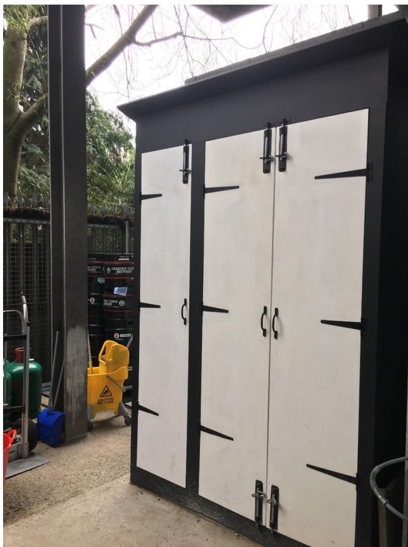
Image 3: View of modern structures to be removed from rear of Arch 55 and replaced with rear extension to match that of neighbouring Arch 56
