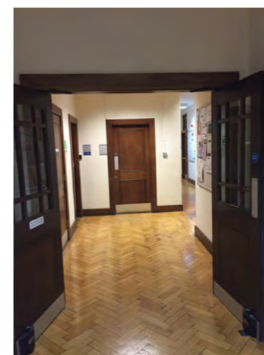
herringbone timber floors, timber windows to stairs and timber doors to be retained / renovated / reinstated in the circulation areas shown in orange.
