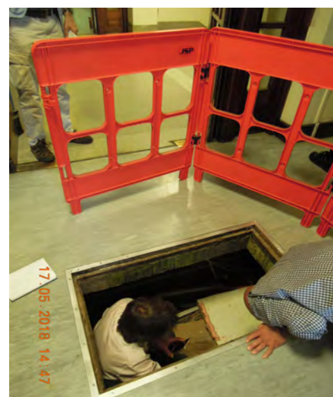
Existing services trench below L3 slab
