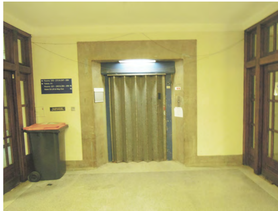
Existing Central wing west stair core - view facing north
