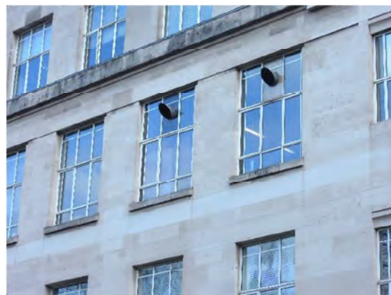
View 34: West Wing façade fenestration
