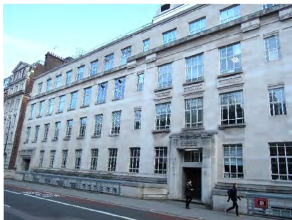
View 33: NW and West Wing façade fenestration
