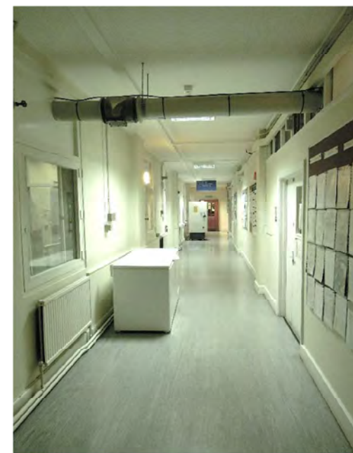
View 17: West Wing L2 corridor facing south
