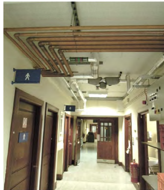
View 30: NW Wing L2 corridor facing south
