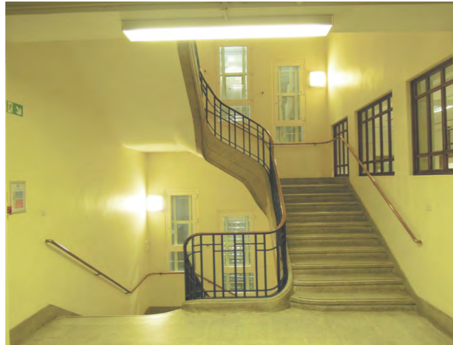
Existing Central wing west stair core - view facing south
