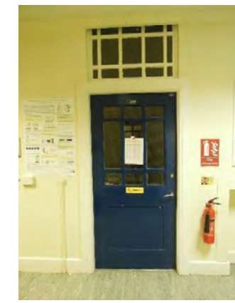
View 12: Central Wing L2 corridor typical door
