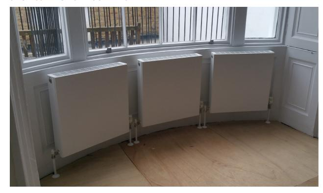
9MS/2/002 Office - As Built Condition with radiators fixed to historical wall panelling / plaster finish
