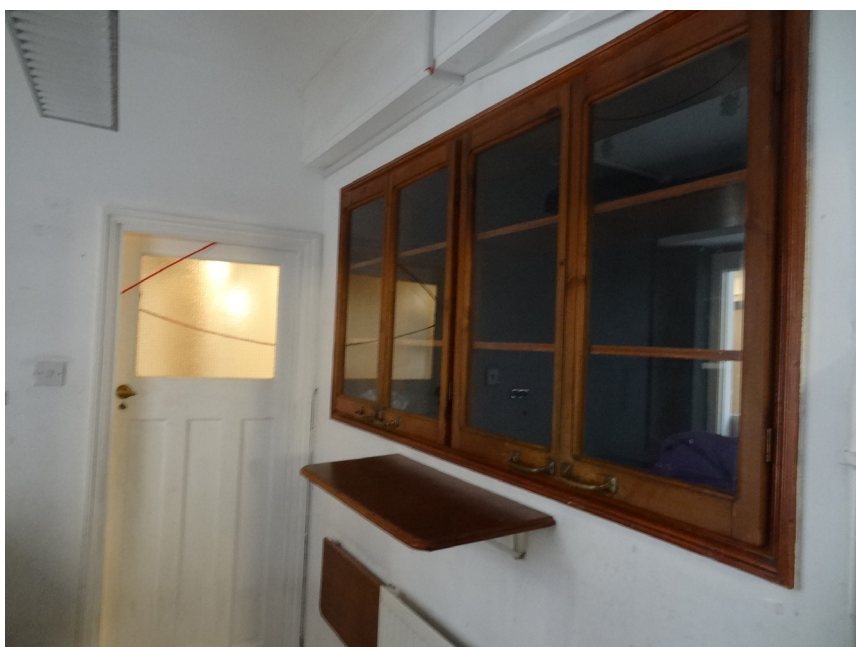
Cupboard in wall and section of wall below to be removed
