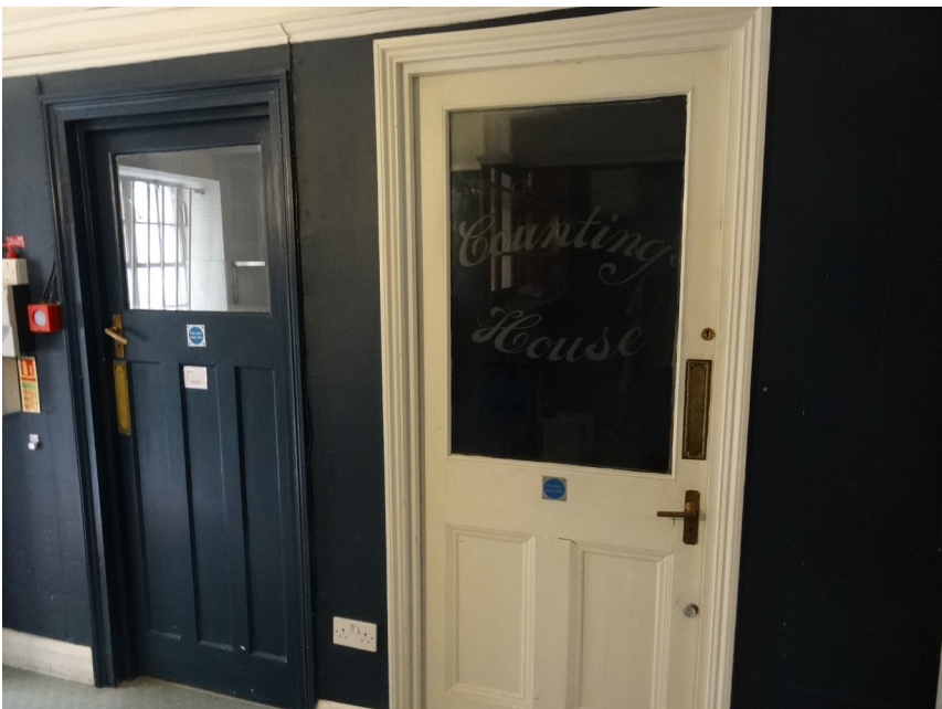
Existing door to Counting Room to be retained as is
