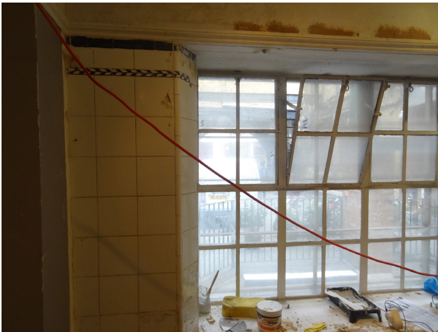
Paint part removed to expose original tiling and detail in G11
