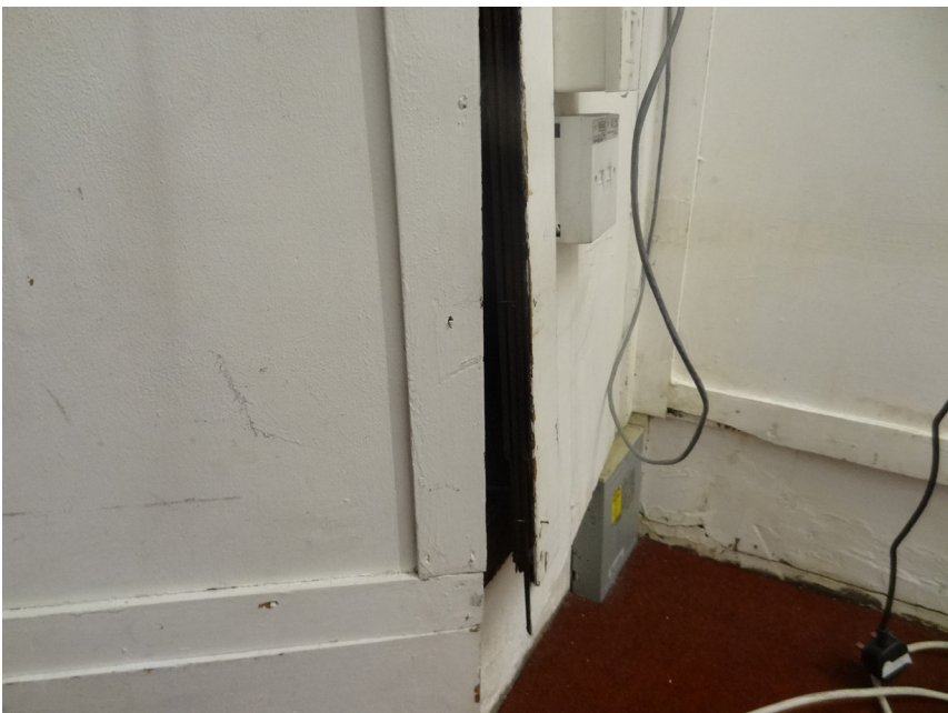
Detail of lower level linings in G4 to be removed
