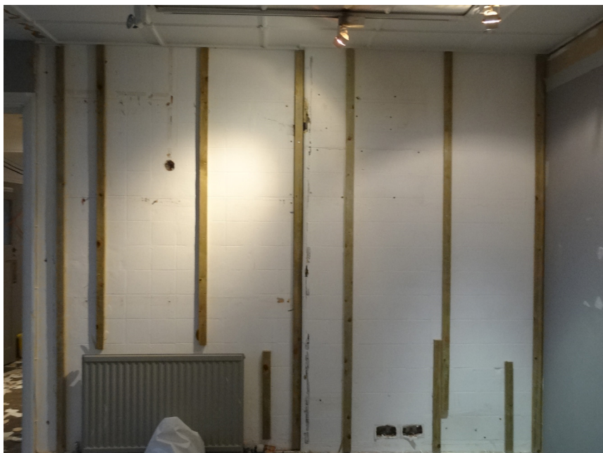
Typical lining battens installed - showing state of wall behind
