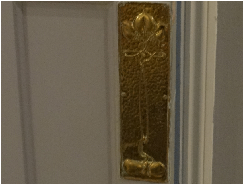
Ironmongery to be retained from door GD07 and reused on door GD08
