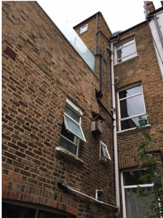
Flat roofed outrigger, with roof terrace, at 146 Iverson Road
