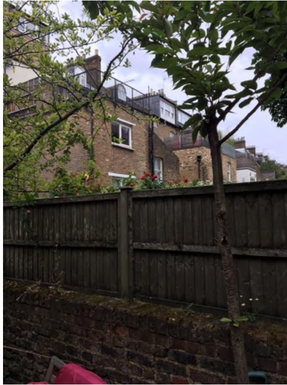
View of flat-roofed outriggers at 152, 156, 158 & 160 Iverson Road
