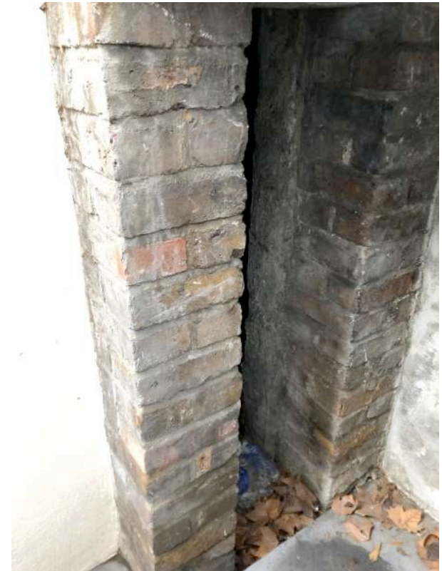
PHOTOGRAPH 03. VIEW OF ENTRANCE TO VAULT
