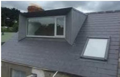
Example of a roof with slate tiles which blend with a rectangular zinc seamed dormer.
