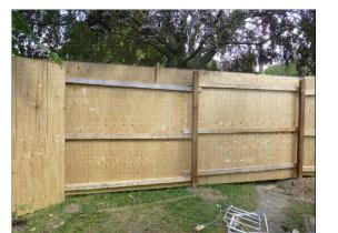
Hoarding to Site Boundary 2.4 m high Timber hoarding fixed to timber posts set at 2.0-3.0 m centres (See Photograph). Where applicable post holes for the timber hoarding will be hand dug using hand held tools and avoiding severance of significant roots of adjacent trees.
