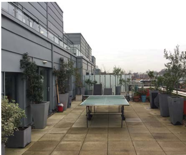
terrace view towards west
