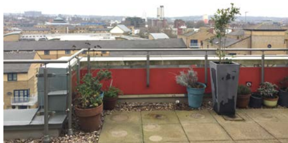
Flat's existing terrace, view towards north
