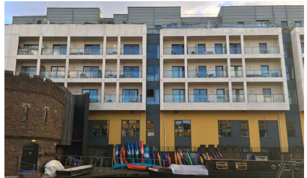
picture of north elevation of Lockhouse building, taken from Regent's Canal
