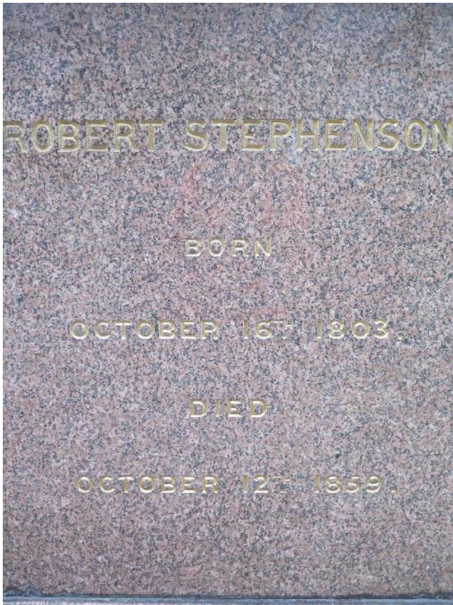
Figure 15 Inscription with letters finished in oil gilding, and below a detail where some loss of gold leaf has occurred revealing traces of the underlying preparatory layers
