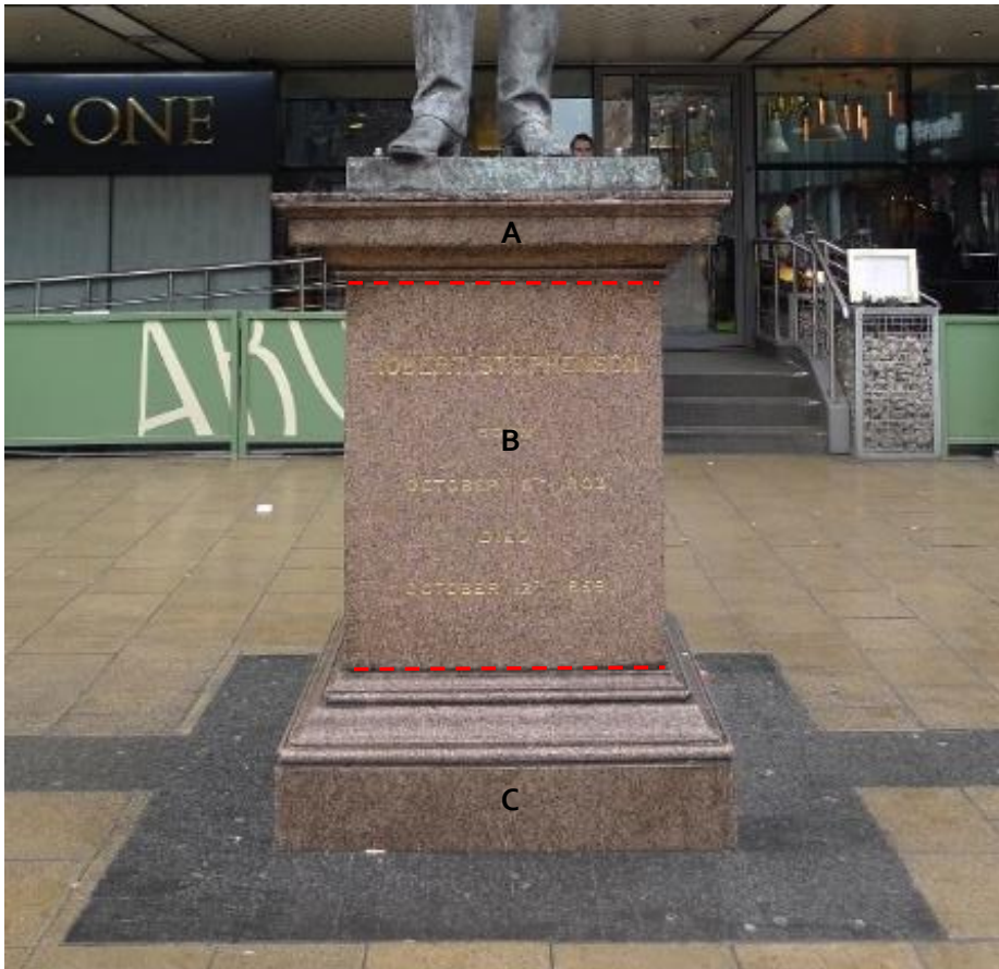
Figure 4 Robert Stephenson sculpture pedestal, facing east, with dashed red lines indicating the fine bed joints between the three pedestal blocks
