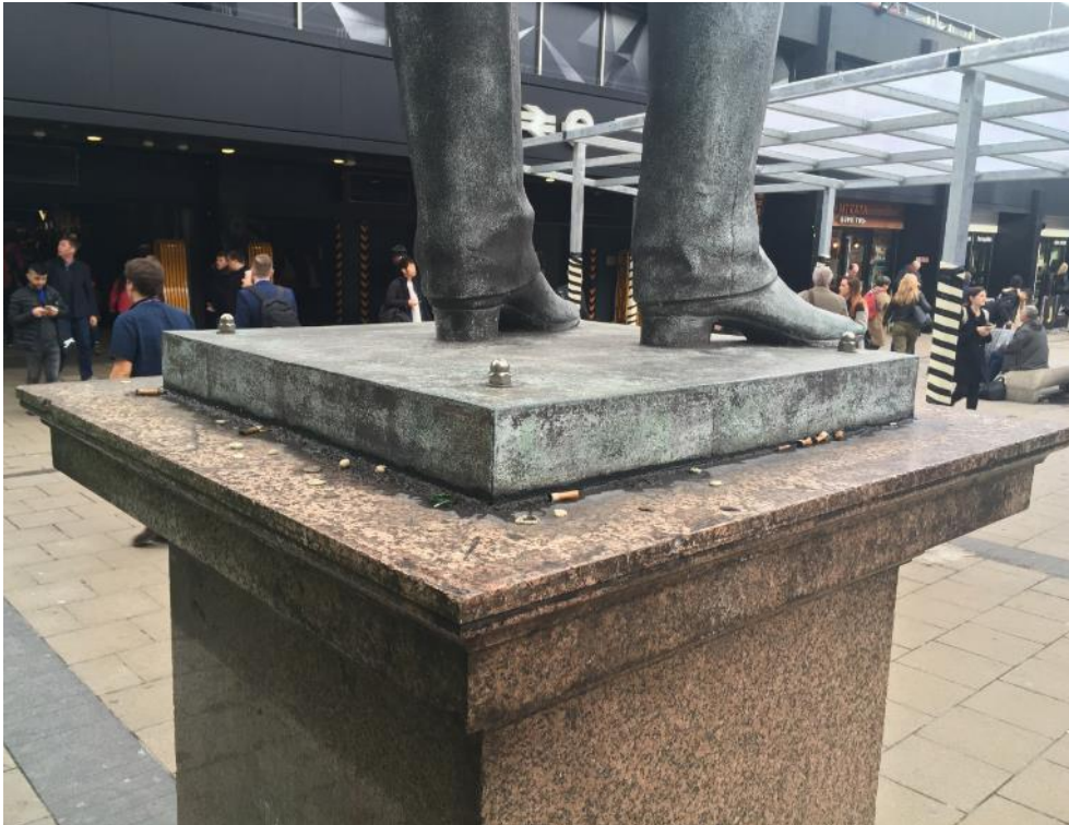
Figure 12 Details of sculpture base illustrating condition and bolts inserted through bronze, with chewing gum on bronze and stone surfaces, and graffiti scratched on the bronze base in image at bottom
