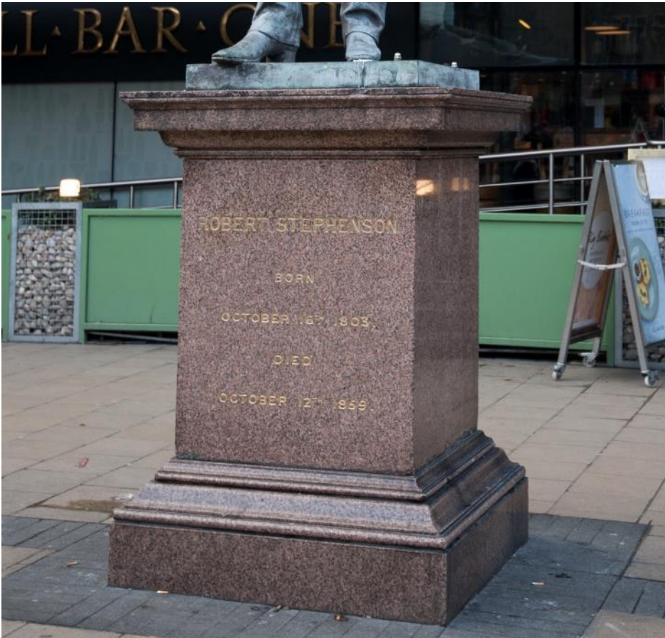
Figure 14 Pedestal from northeast, and below detail of north elevation with dark soiling on base (at lower right) and small spalls along the bed joint, which have been filled
