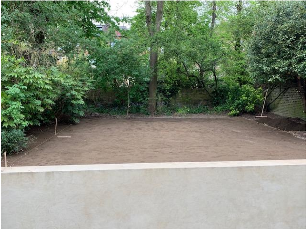
Garden Prior to turf being re-laid.
