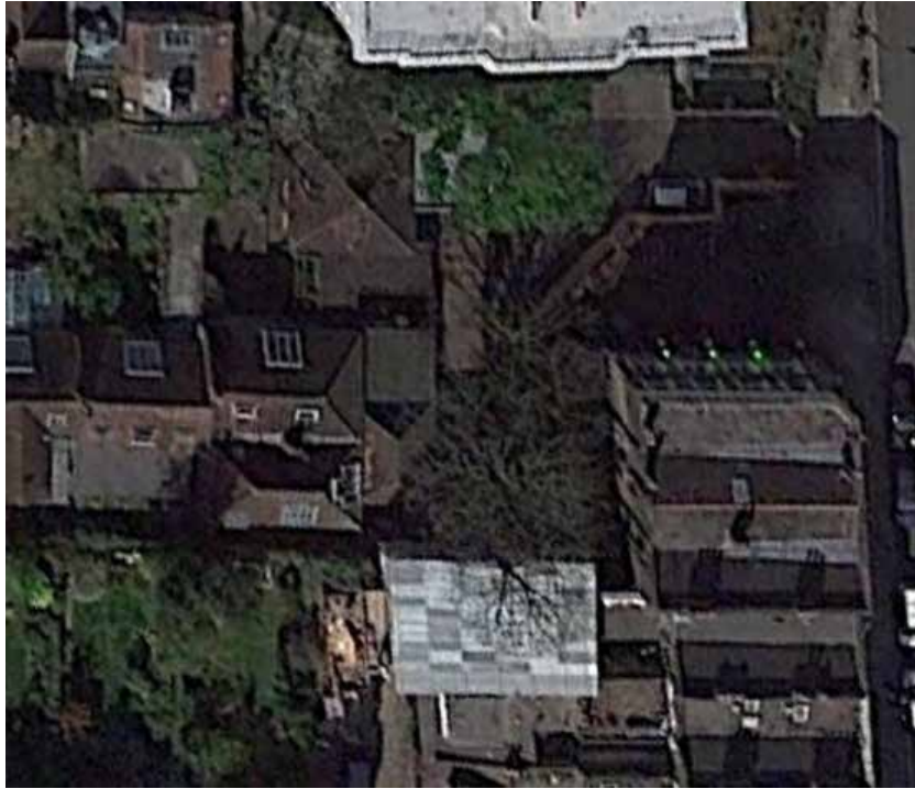
Photograph 1: Aerial view of 1 Steele's Studio, Haverstock Hill, London NW3 4RN (Source: Google Maps)
