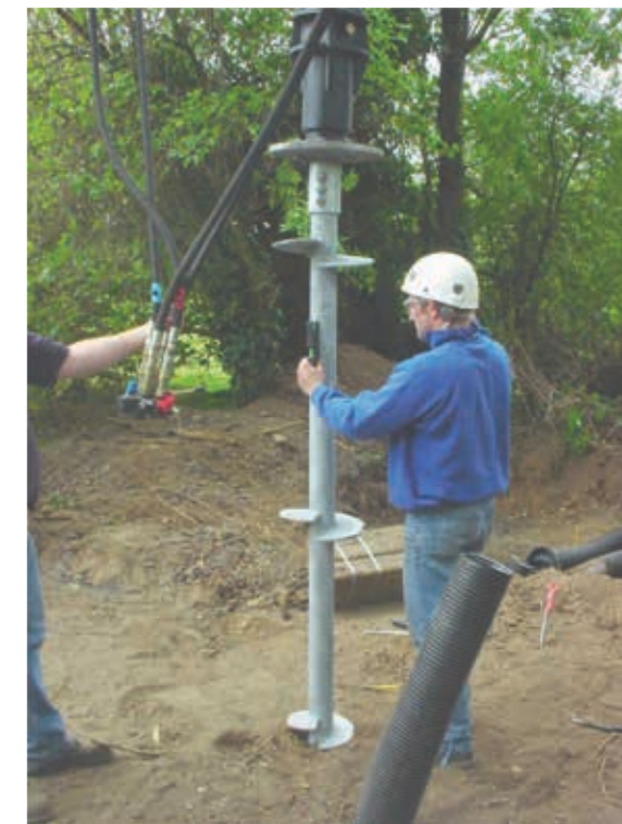
Image of Screw pile installation
