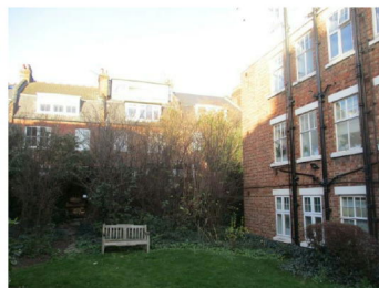
View of trees / shrubs close to area of damage
