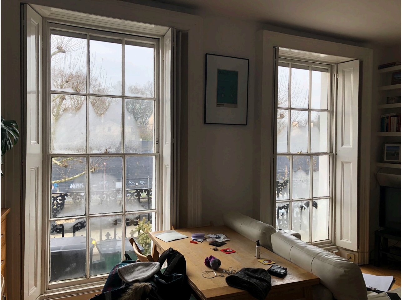
Figure 4: Internal view of windows at first floor (Flat 3)
