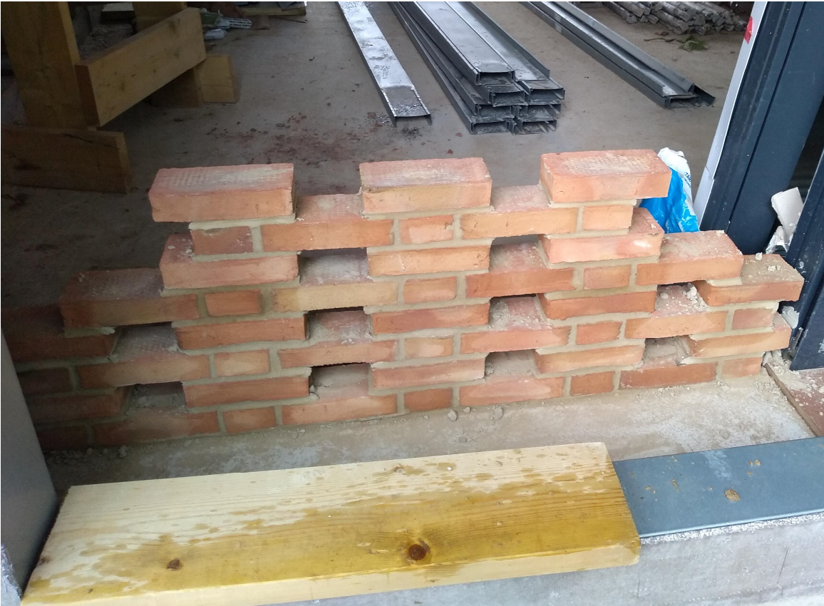
South Façade Brickwork sample panel. Petersen Brick D37
